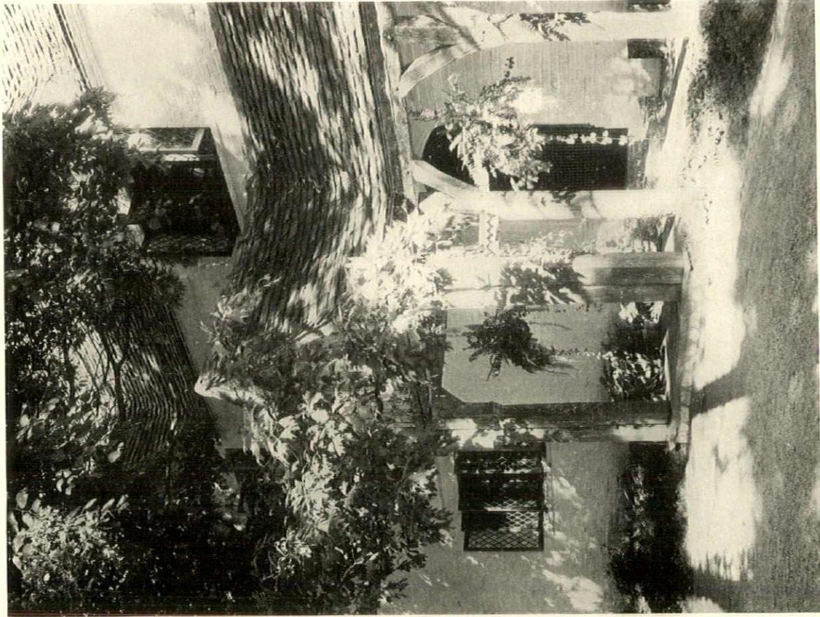
*The main entrance allows of closer examination of the roofing, with its irregular laying and rounded valleys, and shows, as well, the structural integrity of the exterior timberwork*
