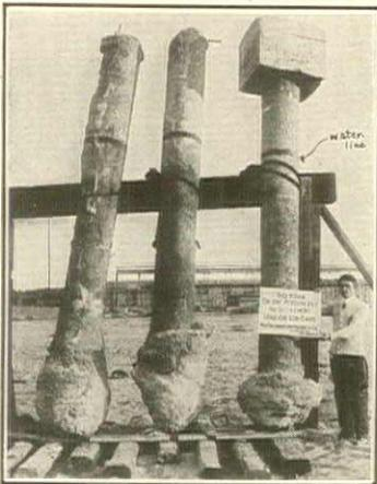
MacARTHUR, Pedestal Type Piles after one of them had supported 50 tons for 10 days without settlement. Note how compressing of concrete has enlarged shaft in pile at left to fill soft spot in soil.
