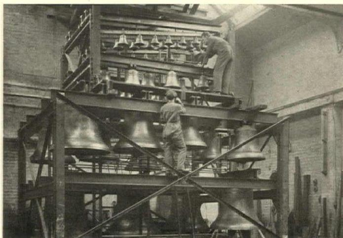
*The bells are mounted upon a steel frame—sixty-three of them in all, covering a range of four octaves*
