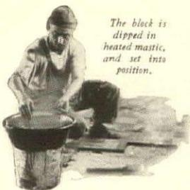
The block is dipped in heated mastic, and set into position.
