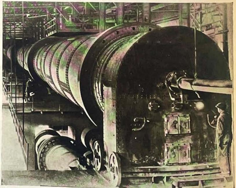
Cement clinker being formed inside this modern rotary kiln at a temperature of from 2,500 to 3,000 degrees Fahrenheit.
