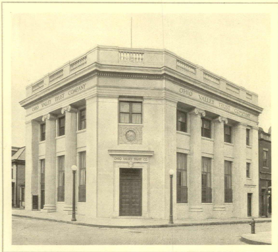
The Ohio Valley Trust Company Building, Coraopolis, Pa. Albert Kahn, Architect. The Foundation Company, General Contractor.
