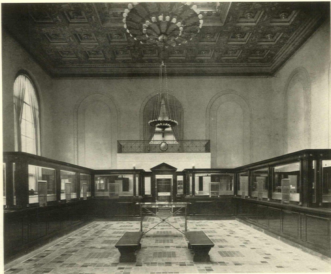
Banking Room, National Manufacturers Bank, Neenah, Wis.
