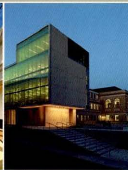
STEVEN L. ANDERSON DESIGN CENTER, UNIVERSITY OF ARKANSAS MARLON BLACKWELL ARCHITECT
