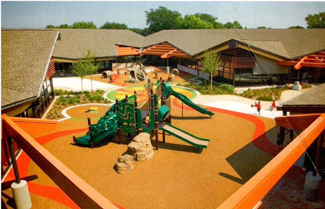
Des Plaines Community Consolidated School District 62, Early Learning Center, Des Plaines, IL | Wight & Company
