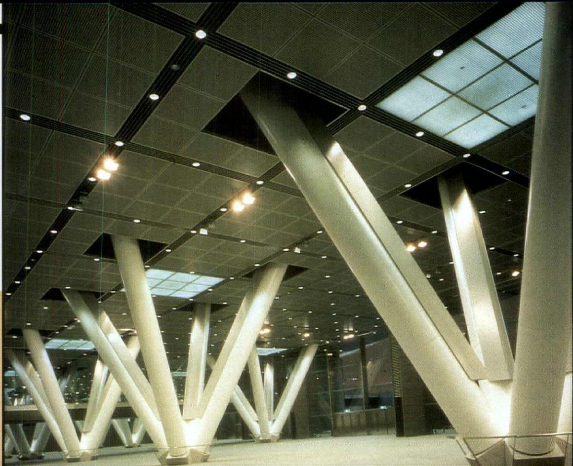
The lighting design for the subterranean exhibition hall (5,000 sq. meters) is also well equipped for diverse activities. Fluorescent lamps are attached at the top of the V-shaped columns, highlighting the structural design, while 150W metal halide downlights and incandescent track fixtures provide more lighting options within the open areas.
