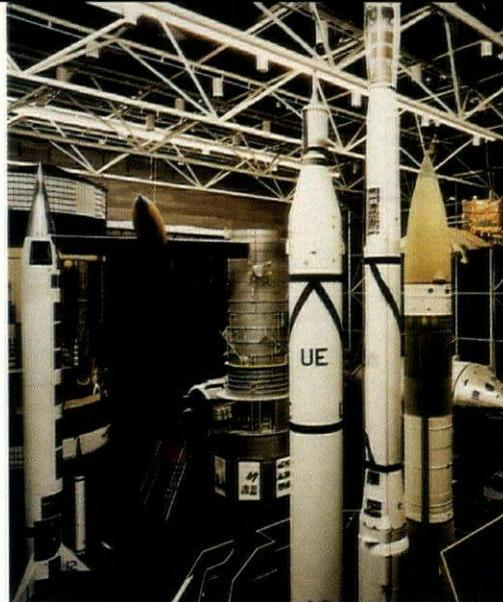
IN A RETROFIT OF A LARGE EXHIBITION GALLERY AT THE NATIONAL AIR AND SPACE MUSEUM IN WASHINGTON, D.C., THREE 90-FT.-LONG LIGHT PIPES, EACH CONNECTED TO A SULFUR LAMP, REPLACED 94 MERCURY VAPOR LAMPS, REDUCING ENERGY COSTS BY 25 PERCENT WHILE INCREASING LIGHT LEVELS BY THREE TIMES.
