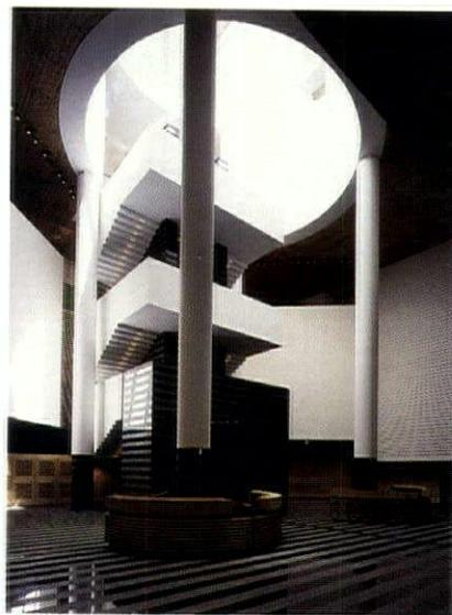
CUSTOM WALL WASHERS, INTEGRATED INTO THE UNDERSIDE OF THE STEPPED CEILING OF THE STAIRCASE, ILLUMINATE THE BANDED STONE WALL, PROVIDING SUFFICIENT ILLUMINATION FOR THE STAIRS (OPPOSITE). THE STAIRS ARE LOCATED IN THE ATRIUM LOBBY OF THE MUSEUM, AN OPEN, DAYLIGHTED SPACE (ABOVE).
