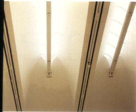
DAYLIGHTING AND ELECTRIC LIGHTING ARE INTEGRATED IN THE GALLERIES (LEFT). DAYLIGHT IS INTRODUCED THROUGH TEXTURED GLASS SKYLIGHTS. BELOW THE SKYLIGHT, A LOUVER, FABRICATED FROM STANDARD STAMPED METAL, ELIMINATES DIRECT SUN. THE DAYLIGHT EXITS TO THE GALLERY THROUGH A GULL-WING DIFFUSER (INSET). IN THE BOARDROOM, A SERIES OF PENDANTS, DESIGNED BY MARIO BOTTA, ARE JOINED TOGETHER TO FORM A SINGLE FIXTURE (LEFT, BOTTOM).
