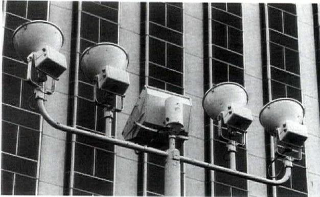
Las Vegas Hilton's new exterior lighting incorporates 175 1,500W Sylvania Metalarc metal halide lamps mounted in five types of narrow-beam fixtures.
