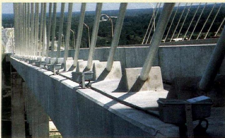
**CABLE READY:** The metal halide lamps are aimed straight up the bridge cables (above, left) at the base of every other cable (above, right). The metal towers are lit with 400- and 1,000-watt halides and 400-watt HPS lamps (below).
