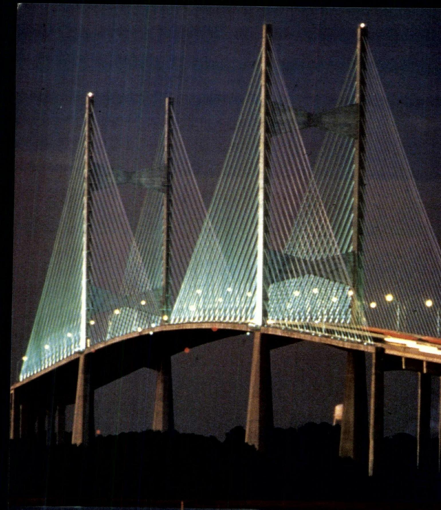
**HIGH & WIDE:** The 400-watt metal halide lamps that were chosen for the Dame Point Bridge project in Jacksonville, FL, feature strong vertical and horizontal beams. The white light brilliantly illuminates the cable stays, which range in length from 6 to 720 feet.
