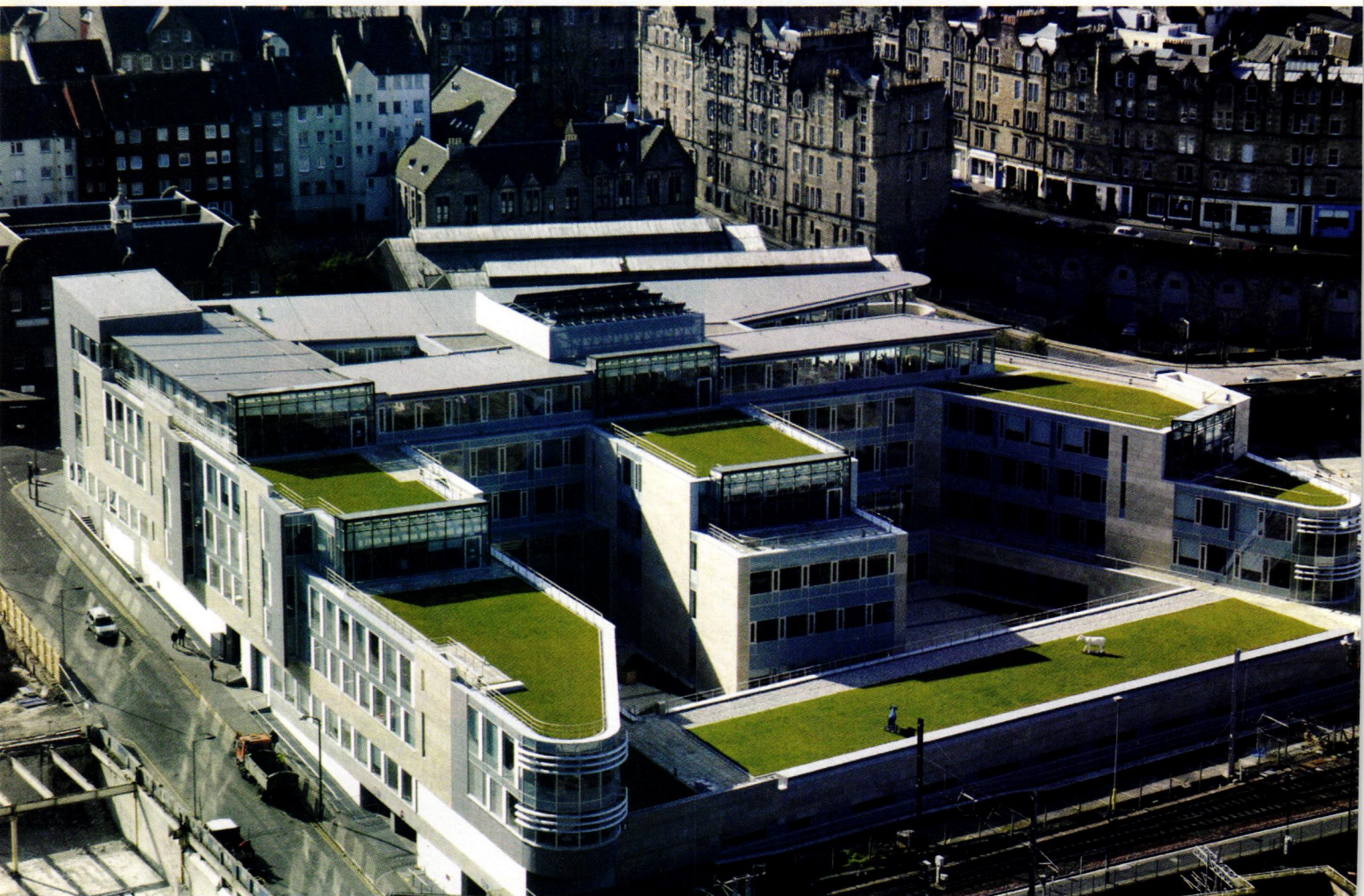
City of Edinburgh Council Offices: ZinCo Green Roof with Hydrotech Waterproofing | Building Design Partnership (Architect) | Briggs Amasco (Roofing Contractor)
