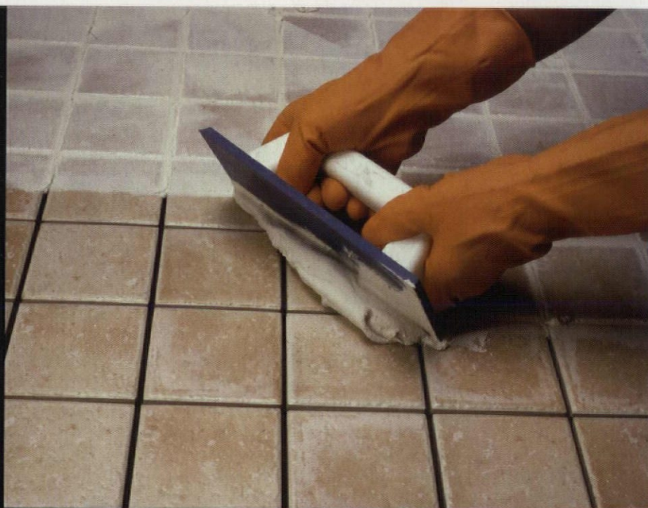
Sealants and adhesives from Mapei play a key role in giving the building its pristine appearance
