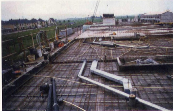
Left: installation of warm-roof panels. Right: pipework will be buried in the screed
