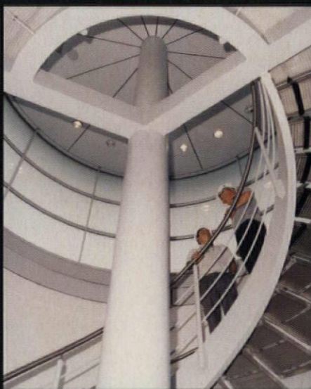
AMEC is responsible not only for the design of M&E but also for its maintenance
