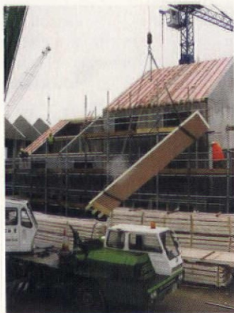
Left: installation of warm-roof panels. Right: pipework will be buried in the screed
