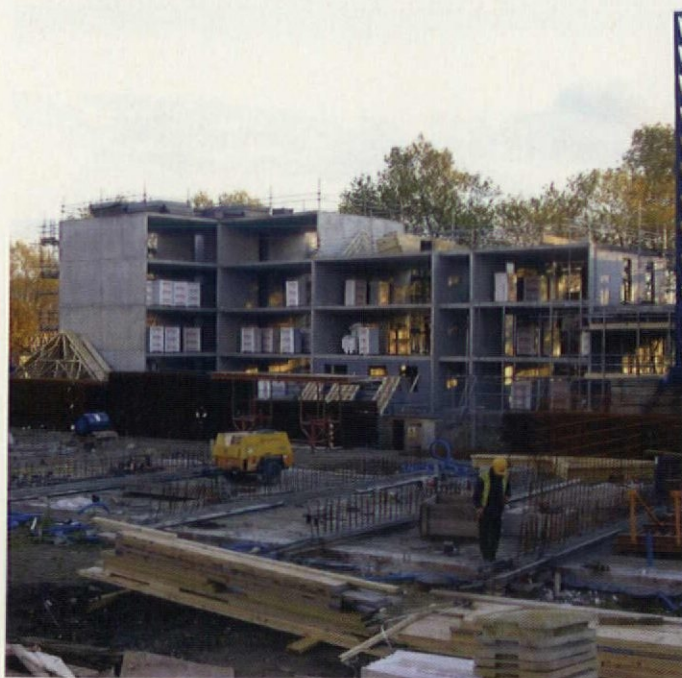
Top: the finished housing at Nightingale will look as if it has been built by conventional means. Above: near-complete housing in the background, and the starter walls in front
