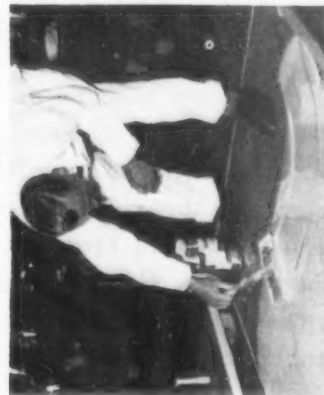
Applying Maximent floor coating
