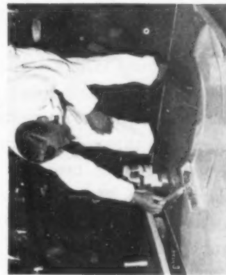
Applying Maximent floor coating
