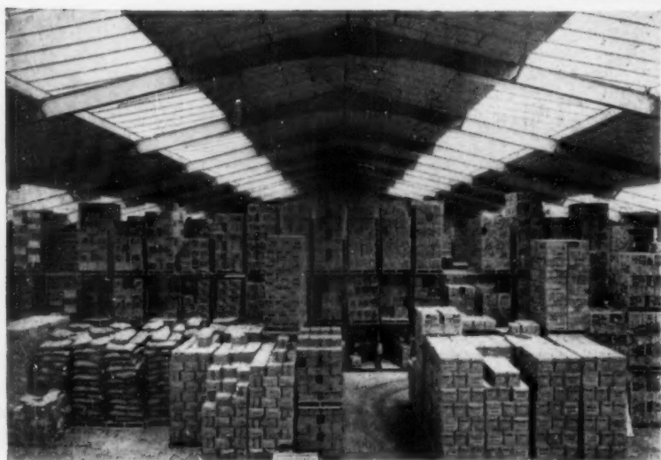
DOUBLE BAY WAREHOUSE Each Bay 100 ft. wide using Portal Trusses to give maximum headroom
