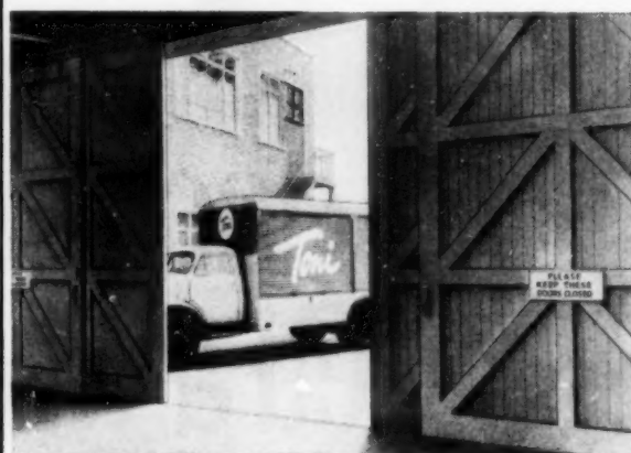
Top hung passing timber doors on Size 4 King Tubuler Track — at the garage of Gillette Industries.
