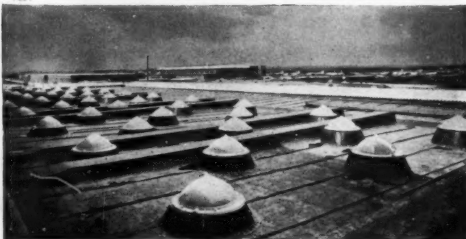
78 domelights made from 'Perspex', 101 sheets of Flat 'Perspex' and 45 sheets of Curved Corrugated 'Perspex' installed on the roof of the Airport Building of 'Brussels National' Belgium, for Regie des Voies Aeriennes.
