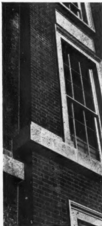
Fig. 1 RUBBA-PAK used on wall sections with column vertical joint.
