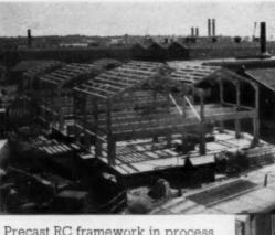
Precast RC framework in process of erection
