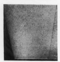
Celotex glass fibre acoustic material on exposed metal fixing
