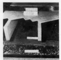
Timber Development Association joist floor supported on ground seal slab
