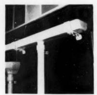
Turner asbestos Slimline gutter
