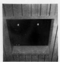
Ruberoid rooflight in galvanised steel decking
