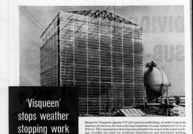
Although these Visqueen shelters were put up by Whessoe Ltd. for specialised construction requirements, they show clearly how effective weather protection can be provided on building projects whether large or small.
