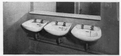
These Standard' Kingston wash basins in one of the cloakrooms at the Ariel Hotel are made from vitreous china. Vitreous china, fired at a far higher temperature than other ware, is more durable and hygienic, and does not rely on its glaze to make it watertight.
