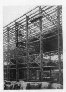
I.C.I. For I.C.I. a Laboratory Block. A multi-storey building with a height to eaves of 4ft. and uninterrupted spans of 50ft. on each floor. Deep Lattice Beams and light stanchions were used with considerable saving in steel requirements.
