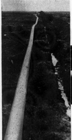
6" 'Polyorc B' p.v.c. pipe made by Yorkshire Imperial Metals Ltd., from 'Corvic' I.C.I. vinyl polymer on site on the Isle of Lewis after jointing and before lowering by hand into its trench. This pipe is part of a 3½ mile water main installation for the Ross and Cromarty C.C. County Water Engineer, G. Peat, Esq., B.Sc., M.I.C.E., M.I.W.E.
