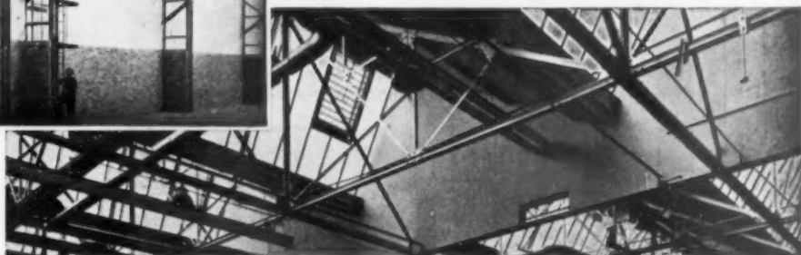
Fire stop in roof truss.
