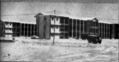
Some 3 storey living quarters. Note the glued laminated timber columns.
