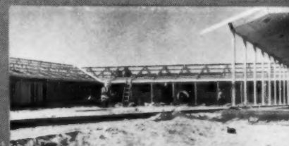
A storage building in Simms Timber construction nearing completion.
