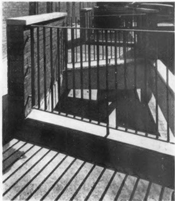
Openings in the ground floor slab to the rear of the shops provide light and air for a car park in the basement
