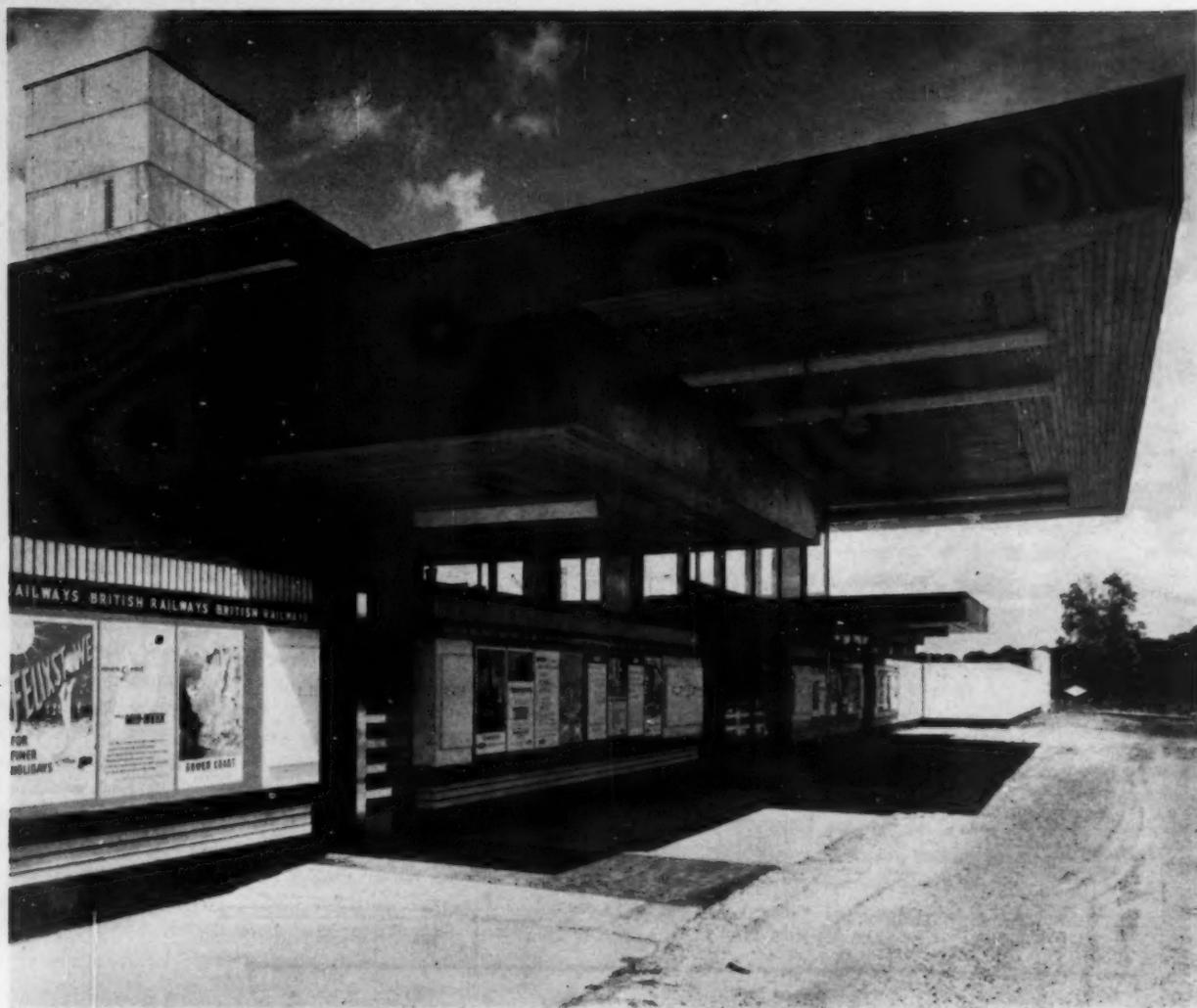
*In essence the station consists of a series of horizontal roof elements separated from each other and the bottom walling by glass or fresh air. At each side of three entrances are massive stone quoins bearing in incised letters of gold the legends CYCLES—CYCLES, HARLOW TOWN—HARLOW TOWN, ENQUIRIES—PARCELS. The linear brass ornament to all doors is well shown in this view*
