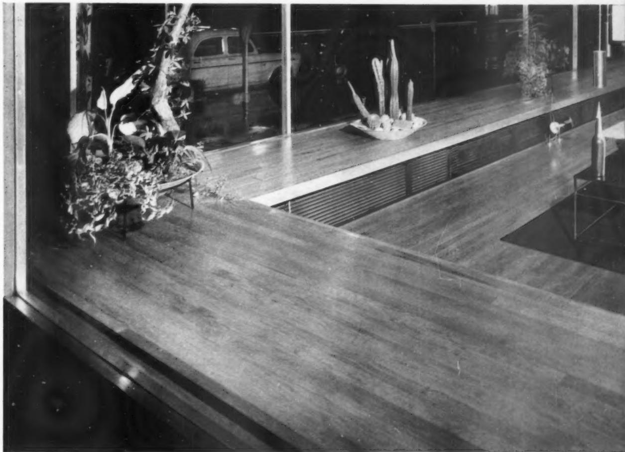
*This afrormosia stallboard is laid on a timber raft which in turn is bolted to a framing of slotted steel angle.*
