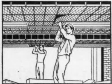
**Expanded Metal is a major economy** Expanded Metal keys are permanent quality keys. With suitable plaster mixes a very high fire rating can be achieved and an exceptional degree of acoustic control attained. These benefits are additional to low initial cost.
