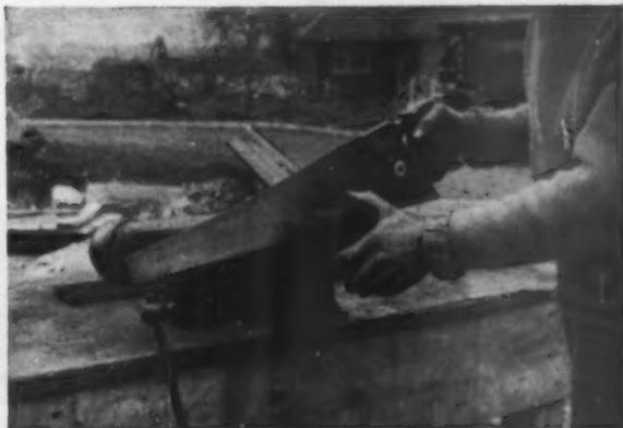
**EASY** to cut. Flexpipe can be sawn to any length as easily as softwood, and there's a specially designed tool for tapering the ends.
