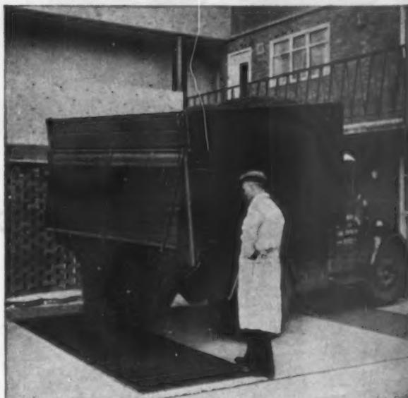
Coal is run simply and quickly through the grate into a hopper below. This hopper holds sufficient anthracite for 2 months' winter consumption. The anthracite is fed by gravity from the hopper into the electrically-driven loader
