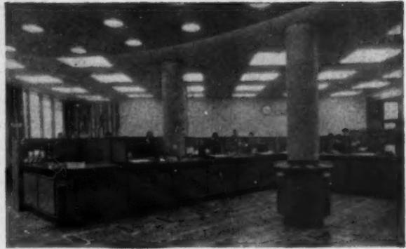
Modular ceiling lighting fittings with opal 'Perspex' diffusing panels made by the General Electric Company Ltd. and installed at the Midland Bank Ltd., High Holborn branch.
