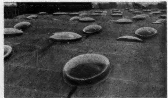
58" diameter Duplus domes made from 'Perspex' by Duplus Domes Ltd., of Leicester. These domes are used on the barrel vault roof of Loughborough College, property of the Leicester County Council.
