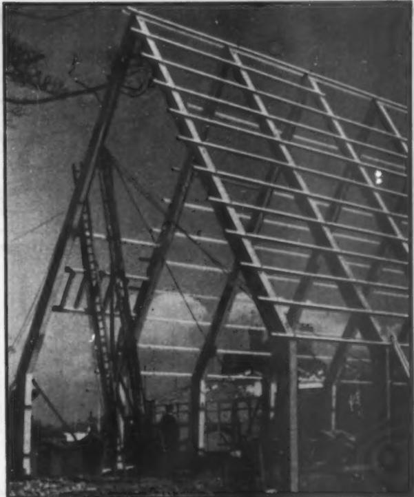
By courtesy of Messrs. Shipley & Foster, Chartd. Archts., we show the Portal Frames to the new Anglican Church at Walsall. Clear Span 34ft. 0in., height to Apex 40ft. 0in. T. G. Construction Co. Ltd.—one of the Tarmac Group of Companies—erected the portals.
