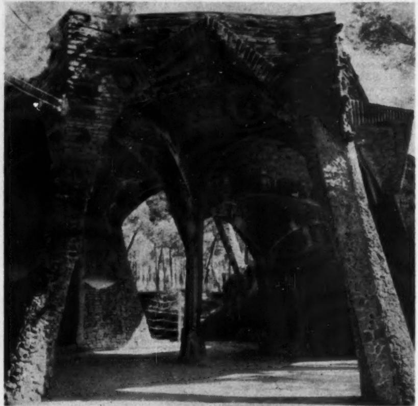
*Flying buttresses were merely crutches to Gaudí, so he hung loads on wires from the ceiling and translated the resulting near-parabolic curves into tilted column structures such as this unfinished chapel in the Parca Güell.*
