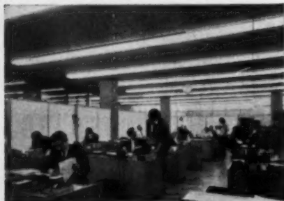
The DAEMPA ceilings throughout Castrol House are fitted with continuous trough cold cathode lighting with diffusers made from diamond pattern 'Perspex' acrylic sheet by Ionlite Limited, Scrubs Lane, London, N.W.10.
