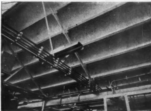
Food factory tongued and grooved timber roof lining sealed against moisture vapour penetration by "PLASTAPAK."
