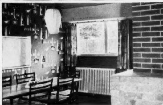
Meals corner is heated by a column radiator under the window.
