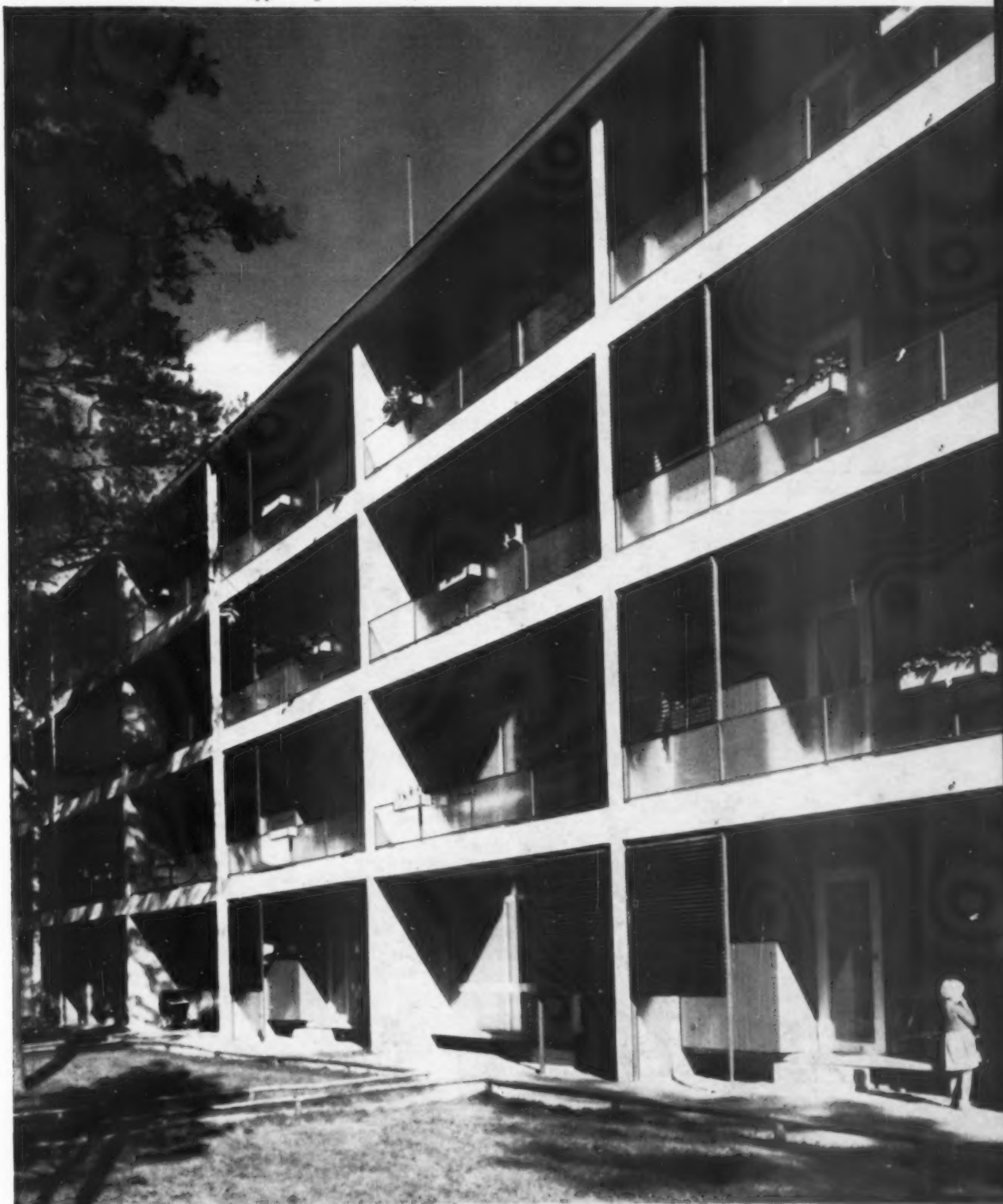
This precast concrete balcony is formed as a tray and is supported at each end on cross walls. Note the projection of a highly-insulated ladder into the balcony space.
