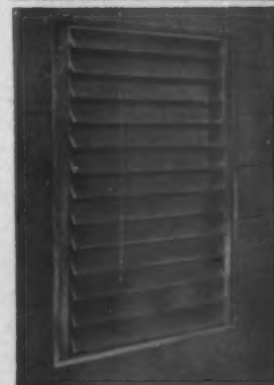
Louvered air inlet ventilators.
