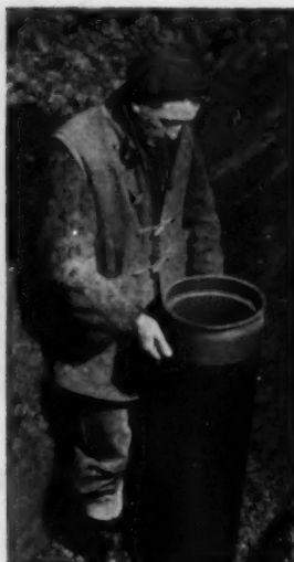
The rubber sleeve is slipped over the spigot end of the pipe.
