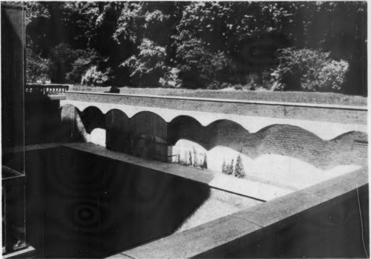
The courtyard behind Weeks Hall. Although this was formed out of the basement of the previous building, the irregular cantilevered arches are new, the soffits taking their form from the original basement vaults which formed the basis for the shuttering
