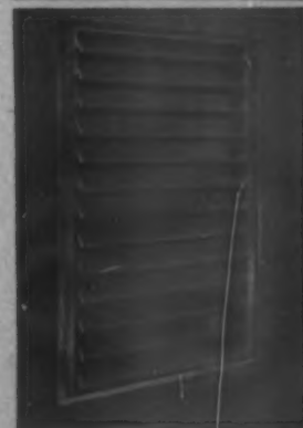
Louvered air inlet ventilators.
