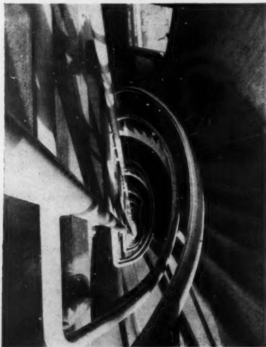
Interior of the elliptical secondary staircases. This staircase, precast in flights and bolted to the in situ concrete landings, is a prototype for the internal set stairs in later blocks. There is a 3-in. gap between the external wall and the stairs. Treads and risers are finished rubber combines, soffit and sides are left smooth concrete
