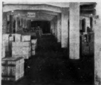
Harbour warehouse, Gothenburg, subject to continuous 4-ton truck traffic. Still in good condition after 8 years, without maintenance.
