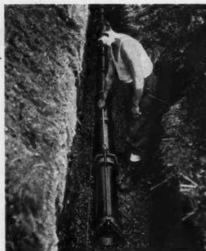
The jointing tool drives the spigot home into the socket.
