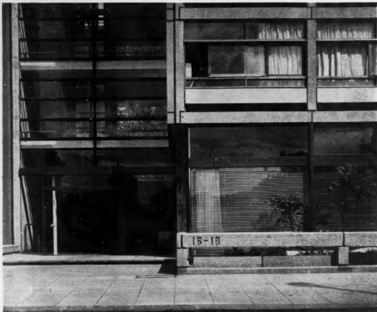
Main entrance. Cornish granite aggregate is used for the precast units to cross-walls and edge-beams, white Norwegian quartz to study-bedroom under-window panels. Study-bedroom windows are untreated Burma teak. Metal windows are painted dark blue-grey. All curtains are lined
