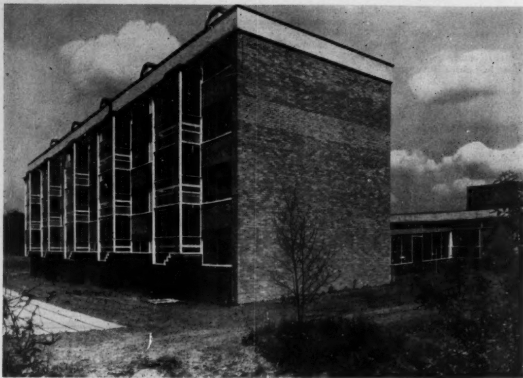
The cantilevered landings and stairs to bedroom floors of the night unit
