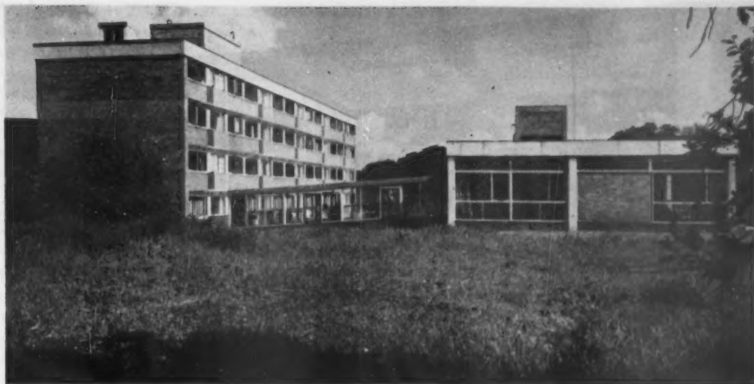
The linking corridor between the day and night units follows the natural slope of the ground. Glazed areas are much reduced in the night unit
