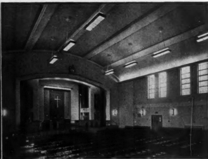
Lighting units, each weighing over 2 cwt., are serviced by means of L.E.F. Raising & Lowering Gear at the Leysian Mission Hall.
