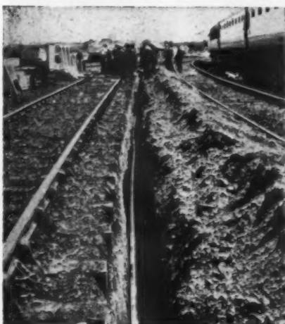
Corrosion resistant 'Chemidus' 2" pipe made from 'Corvic' vinyl polymer lowered into its trench after jointing at new carriage sidings near Vauxhall Station, Great Yarmouth. The pipe was made by Chemidus Plastics Limited, Progress Way, Purley Way, Croydon, for British Railways, Eastern Region.
