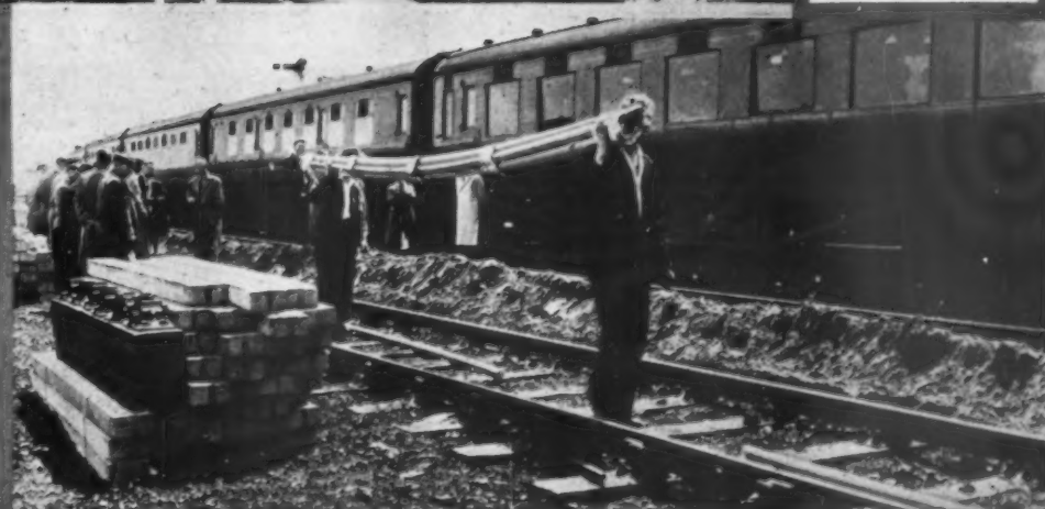
Four 20 foot lengths of Chemidus pipe being carried on to the site.
