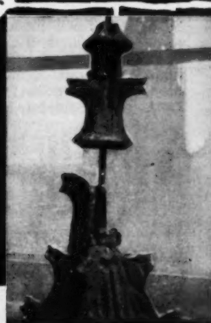
Cap of pinnacle at Houses of Parliament split by corrosion of iron centre rod (afterwards replaced with "Delta" Bronze No. IV).
