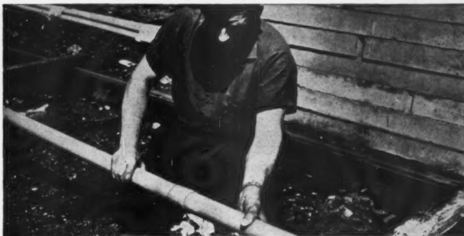
Joining Chemidus pipe by means of a special cemented socket and spigot joint developed by Chemidus Plastics Limited.
