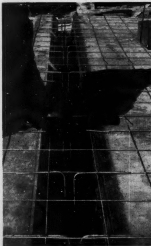
Preparing reinforcements in moulds. The steel is galvanised to minimise risk of staining from rust
