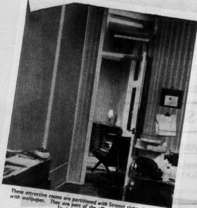
Stramit slabs in timber framing at the offices of Midland Electricity Board, Kingswinford, Worcs.
