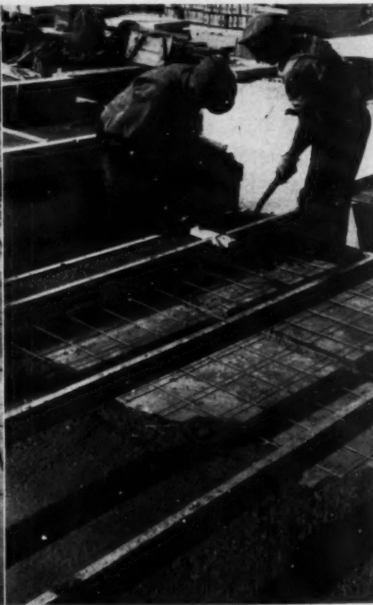
Laying in and vibrating the ordinary Portland cement concrete which forms ribs and backing to slabs
