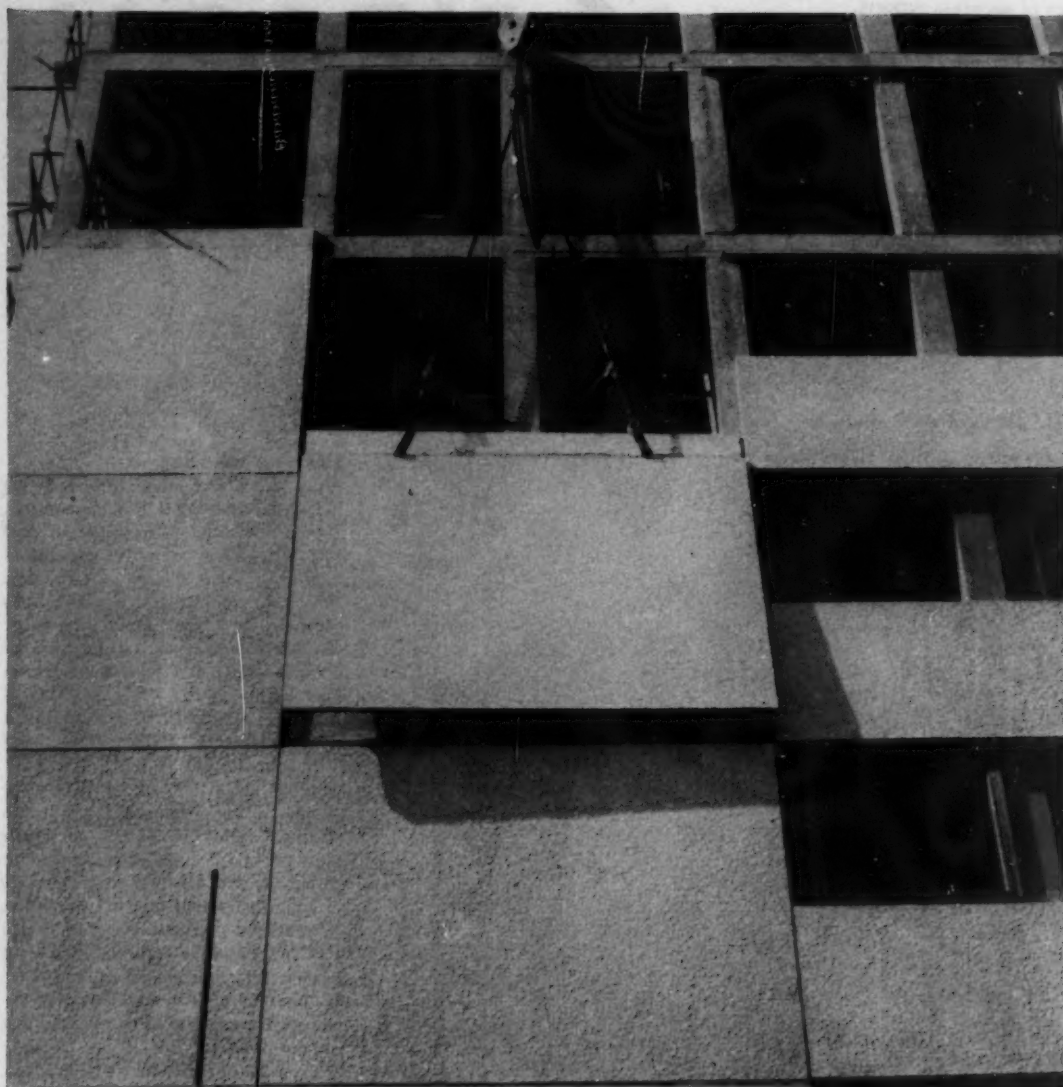
Lifting a cladding slab into position
