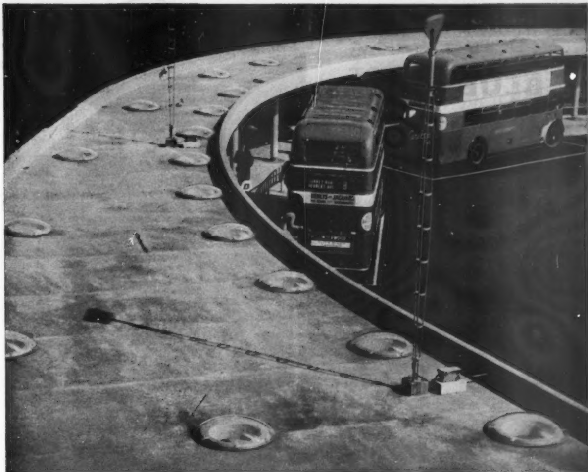
100 'Duplus' Domelights made from 'Perspex' acrylic sheet by Duplus Domes Ltd., Chatham Street, Leicester, are installed on the roof of the Bournemouth Bus Station of the Hants and Dorset Motor Services Limited. Architect: Alan A. Briggs, F.R.I.B.A., The Tilling Association Limited.
