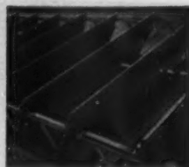
Roof ventilating shutters.
