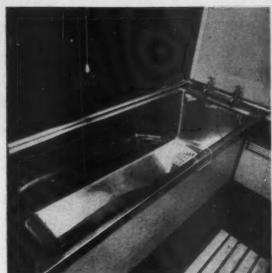
For economy and hard wear special stainless steel baths were made. On the wall is the emergency signal.
