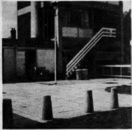
Service area: a business-like space, marred only by the lack of storage for bins and rubbish. External doors are aluminium-faced, opaque panels are plastic-bonded glass.
