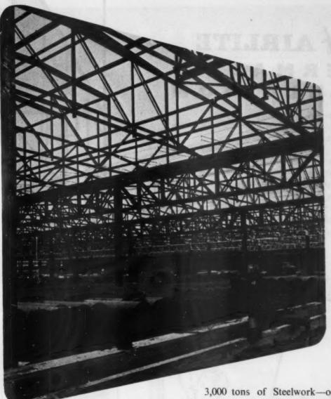
3,000 tons of Steelwork-of welded construction throughout-for a new factory in South Wales for the Prestcold Division of the Pressed Steel Co., Ltd. The whole framework was erected within six months!
