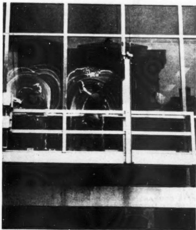
Fig. 10. Lever Building windows being cleaned from cradle.
