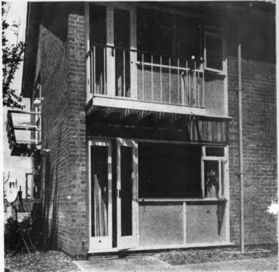
Metal and timber balcony balustrades on adjoining faces of the south corner of Grenfell Hall.
