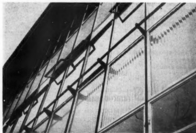
Fig. 5. Rail for ladders, Oldwood County School, Manchester (Manchester City Architect).
