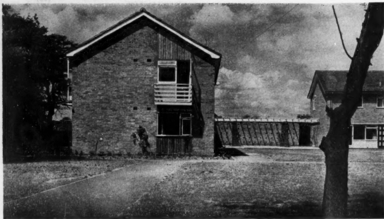
Gable wall, block A (ground floor plan on page 442). Mahogany boarding, white-painted timber balustrade on balcony.
