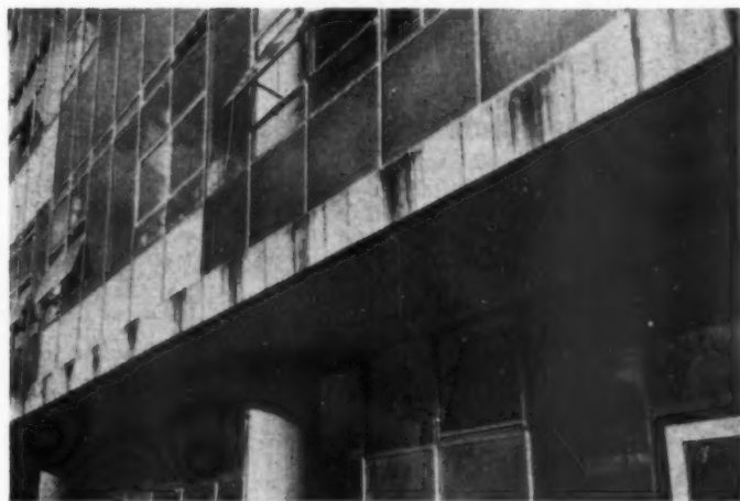
Fig. 4. Copper staining, Tulse Hill School.
