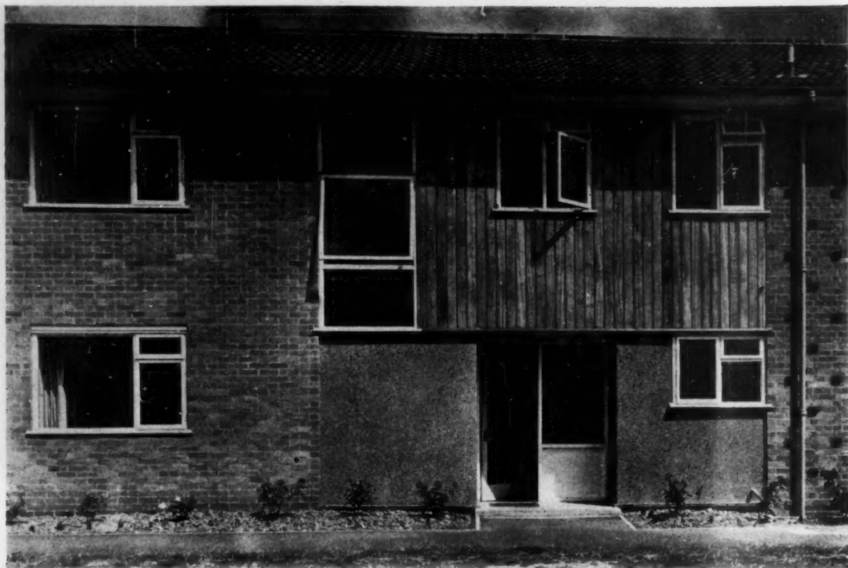
Entrance to a staircase unit. Mahogany boarding to first floor and self-coloured rendering to ground floor.
