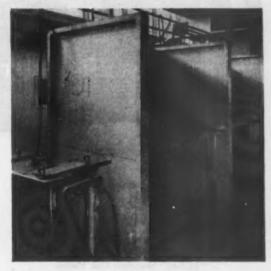
The cubicles for arc welding (232). This is not a successful layout, as may be diagnosed from the dangerous arrangement of cables and the indifferently rigged conduits. The shortcomings arose from an inadequate appreciation of the services-to-equipment problem.
