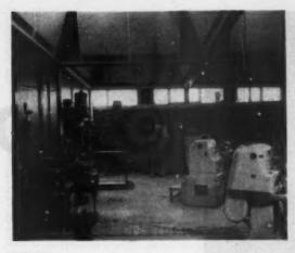
The Machine Shop showing the drilling machines against the wall on the left and some of the centrally sited lathes (202). Note flexible conduits to overhead bus-bars, the store in the background and the heater units at high level.
