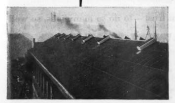
Exhaust gases from fork lift trucks and lorries were once a major problem in this storage shed. Colt experts were called in to make a scientific analysis and on their recommendation a series of Colt S.R.C./3090 High Duty Extract Ventilators was installed. Fumes no longer bother anyone.
