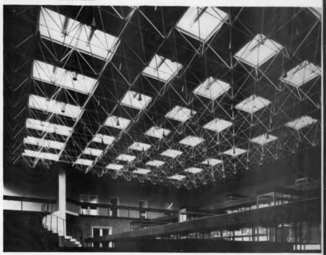
This space frame made up of tube, rod and angle, is based on a module 4 ft. 0 in. square to which woodwool slabe and rooflights of standard dimensions are related.
