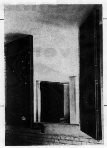
An installation of a Mather & Platt self-closing, folding armoured fire door, with rising hinges in a factory producing drawing office equipment. In the background is an armoured, sliding door.
