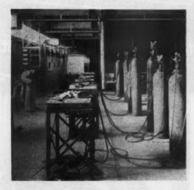
Gas welding benches (233) in the foreground and the arc welding cubicles (232) in the background. Note the neat arrangement of electrical switch gear on the panel on the left at the end of the cubicles. All gear is laid out in this way on special panels to avoid fixture on demountable partitions. (This was carried out under the personal supervision of the architect on site.)
