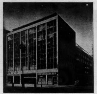
OMNIA Concrete Floors installed in the ATV Headquarters building at the remarkable rate of 9,000 square feet every 10 days.
