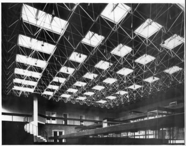
This space frame made up of tube, rod and angle, is based on a module 4 ft. 0 in, square to which woodwool slabs and rooflights of standard dimensions are related.
