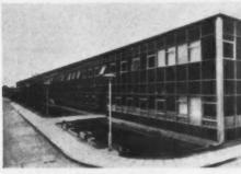
WILLIAMS & WILLIAMS LTD "Wallspan" aluminium curtain walling was selected for the Administration Block of Ford Motor Company's new Spares Division because of the low maintenance cost.
