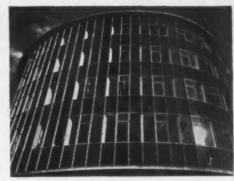
Tower House, Hopton Street, S.E.1, is the first example of "Wallspan" curtain walling being used in a curve.
