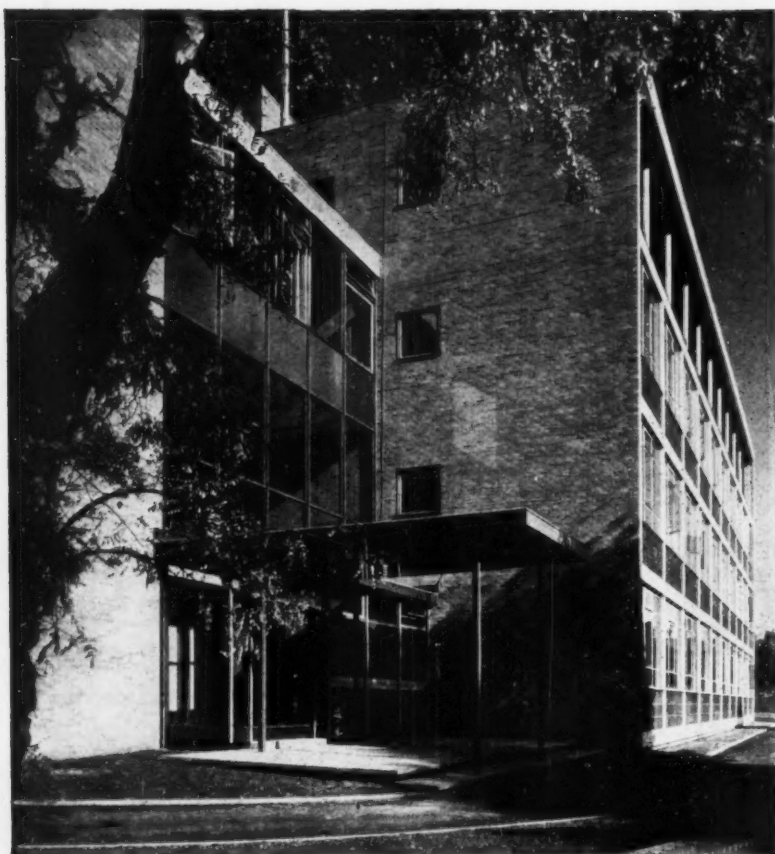
'PLYGLASS' Clear, Diffusing, and Lettered Double-Glazing Units have been used throughout the new office block for the Cambridge Instrument Company Ltd. Architects Edward D. Mills & Partners. Illustrations reproduced by permission of 'Architect & Building News'.
