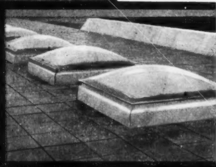
Purpose made continuous base of lights with full visible fabricated ends. This is the latest Cox roof light, specially designed for the Princess Margaret Hospital.
