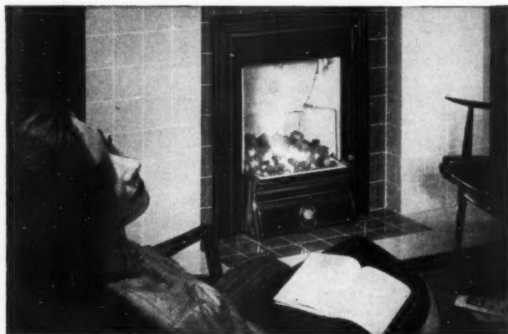
(Left). Installed with Chevin C Inset Fire and Interior Frame No. 37 (used only when convected warm air is returned to the same room).
