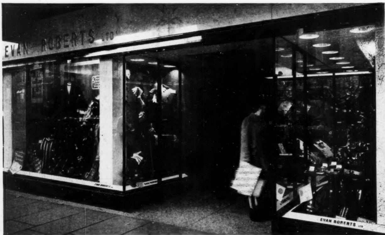
The shop windows were designed by the architects and executed by shop-fitting sub-contractors. The fascia is a white marble with gilt lettering; the skirting is polished blue pearl granite. The revolving door is part of the old, demolished shop, rejuvenated and re-erected.
