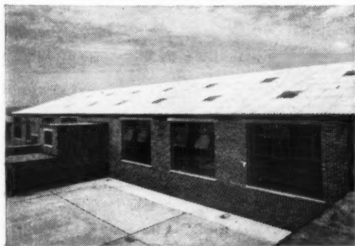
'Arcon' 66 ft. 8 in. span factory building supplied by Taylor Woodrow (Arcon) Ltd., for Bush Radio Limited, Plymouth, in which Clear Corrugated 'Perspex' sheet, type 568 has been used for the roof lighting. Architects: Fuller, Hall & Foulsham.
