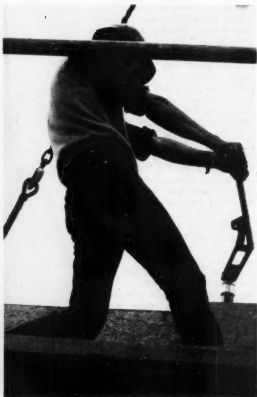
Torsion wrench breaking at predetermined tension.
