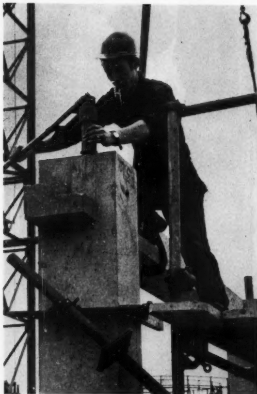
Pre-loading columns by torsion wrench.
