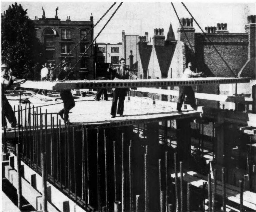
Pre-cast floor slab, showing the transverse holes which reduce the weight.
