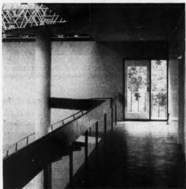
The suspended ceiling around two sides is slightly strange, but acceptable; its junction with the column of the staircase is most regrettable.
