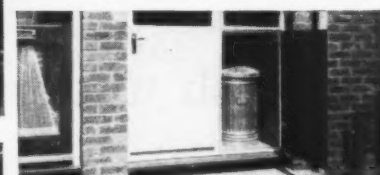
A new way with dustbins Standard equipment throughout Crawley are these dustbin units. The louvred steel front opens on to a steel box which has a hinged lid and contains the dustbin. Rubbish is disposed of from inside the kitchen and collected from outside the house. Specially designed and made for the Crawley Development Corporation by Williams & Williams.
