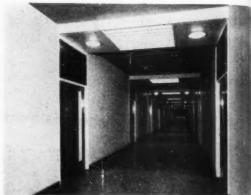
Central corridor in teaching laboratory block. Note the careful detailing by which doors, artificial and natural daylighting are combined into clearly defined units at regular intervals.
