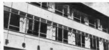
Curtain Walling on the Post Office Williams & Williams curtain walling with yellow in-fill panels give a light, bright look to the new Post Office, situated just outside the Town Centre.
