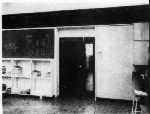
The teaching laboratory: the inside of this block has been carefully considered and is very successful. Note the heat grilles and the glazed side frame to the door, which can be opened for access for bulky equipment.
