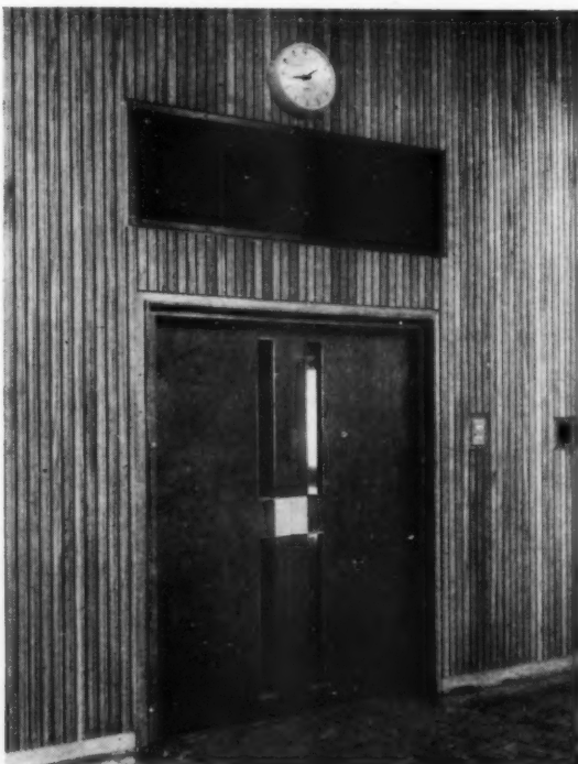
Detail of door into lecture theatre, showing the excellent detailing of the knuckle boards and their cutting around ventgrille, architrave, and light switch.
