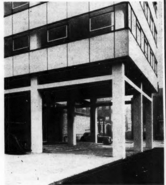
The main entrance to the tower block, which is raised on stilts at this point. The intersecting planes and the horizontal r.c. subframe which corrects the scale of the otherwise spindly pilotti have been cleanly resolved. The forecourt is not yet finished.
