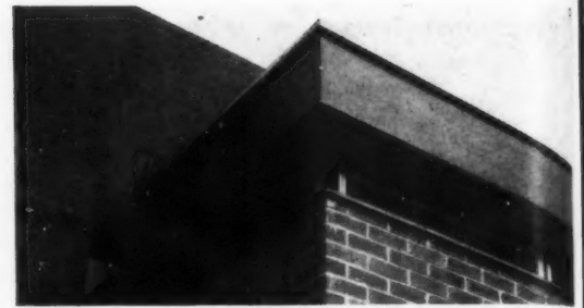
Detail of the exposed r.c. frame over the research laboratories. The felt upstands to the beam look unsightly on some of the frames.
