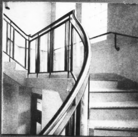
Bronze Balustrading at British Challenge Glazing Co., Stratford High Street, London
