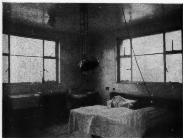
The walls and ceiling of the labour ward of a maternity hospital, shown in the above illustration, have been treated with "Plastapak" to provide a washable aseptic coating.
