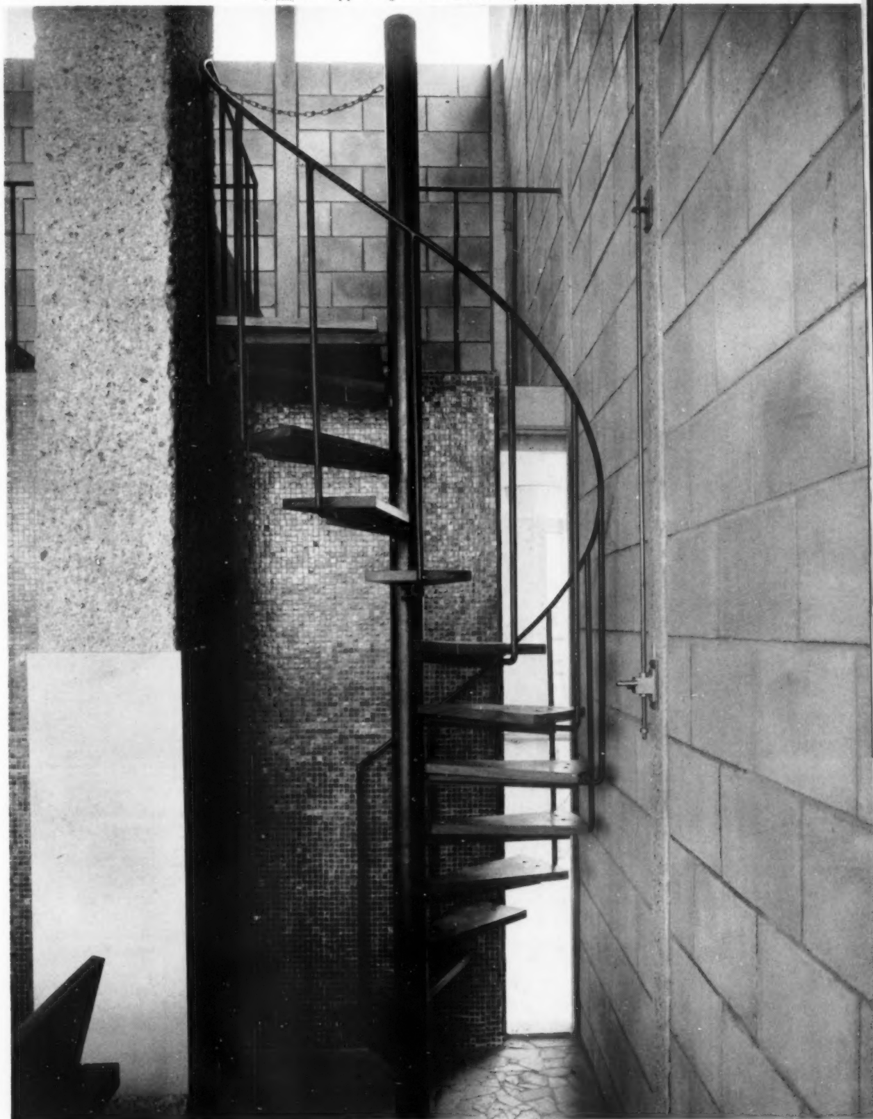
This is an exceptionally neat version of the iron circular stair. Note the iron bracket plates sunk into the underside of hardwood treads (visible in the drawing only) and the termination of the handrail at the bottom in the lowest tread.
