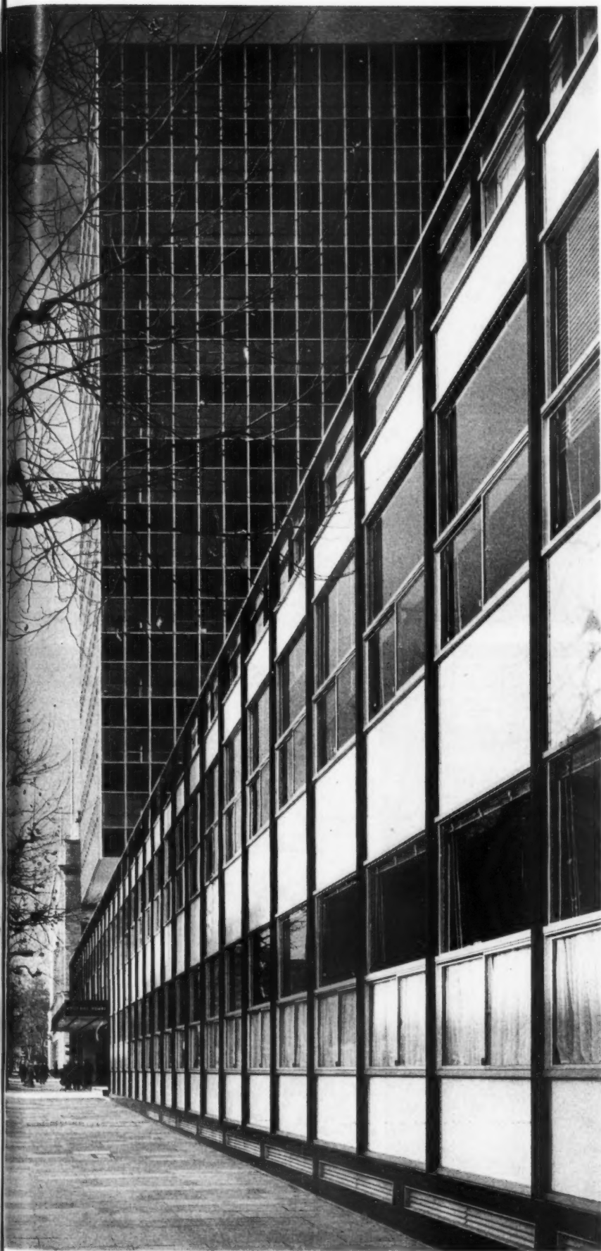
Left: looking along the Marylebone Road front towards the tower and entrance. The spandrel panels are white Sicilian marble. Below: corner of the third storey of the lower block.
