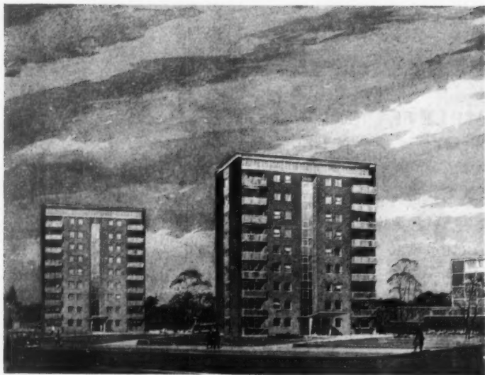
Fig. 1. A perspective of the nine-storey flats. The projecting balconies have wired glass spandrels and the recessed panels between windows on the end elevations are precast exposed aggregate.
