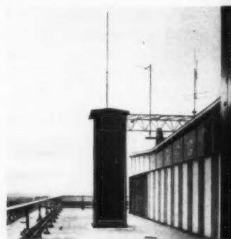
On the roof of the tower block, a successful attempt has been made to initiate some order into an unavoidable proliferation of tanks, ventilation plant, fume cupboard extracts, lift motor rooms and aerials. Here the "sentry box" houses a fume cupboard extract fan and roofhouse to right contains cisterns, lift motors, air conditioning plant for chemistry department, and supports a space frame for TV and radio aerials. White and grey asbestos cement sheet cladding.
