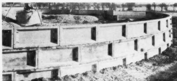
Croft Precast concrete filter bed units are quick to erect and require no skilled labour.
