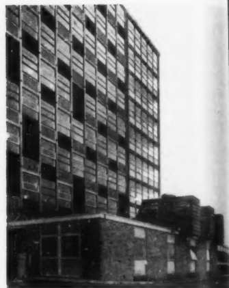
The tower block from the north west, with single storey kitchen and dining hall projecting in front. The under-sill cladding in the centre of the tower is in exposed aggregate slabs in two colours, at the ends in opaque coloured glass. The full-height solid panels which take some partitions at an intermediate point between the frames, are surprisingly unobtrusive and give a pleasant random-ness.
