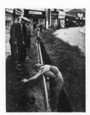
Water main made from 'Corvic'; the bend in the street was negotiated without the use of 'specials' as there was sufficient elasticity to allow for the fairly long-radius bends without any preforming of the pipe.
