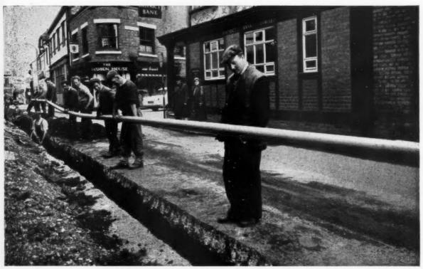
Water main made from 'Corvic' vinyl polymers by Chemidus Plastics Limited, Croydon, being laid already jointed by Mid and South East Cheshire Water Board, Engineer and Manager: Delwyn Davies, M.I.C.E., M.I.W.E.
