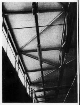
A closer view of the overhead arrangement of fluorescent lights and radiant heaters, each running in lines at 12-ft. centres, 6 ft. apart. Above each single line of high temperature high pressure hot water pipe can be seen the insulated metal reflector units radiating the heat downwards.
