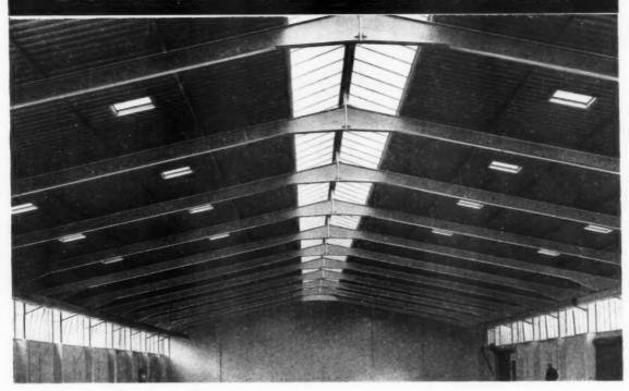
Warehouse, 100ft. span. Roof Pitch 12°. Alford & Alder (Engineers) Ltd.
