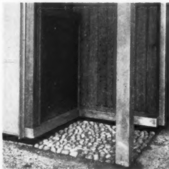
Below left: At corner stanchions in the administration and laboratory block the cladding is set back. Infilling includes asbestos cement panels, beaded in, and vertical cedar boarding, the latter being shop fabricated into panels requiring fixing only. The perimeter paving of the building is generally exposed aggregate concrete with cobbles infilling areas when the cladding has been set back. Below right: in the same position, the column head is exposed, showing the assembly of the main members of the aluminium frame.
