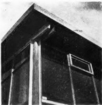
Above left: cladding is carried in vertical aluminium tees, here in the test shops, at 2 ft. 8 in. centres. At corners these are fixed to 4 in. by 4 in. timber posts. The top chord of the aluminium portal frames, formed of two channels, oversails to carry the eaves. Above right: at the footings, tees and cladding have been carried down beyond finished floor level, but the 4 in. by 4 in. post sits on the site slab with aluminium flashing below. To avoid unnecessary delays in construction, 4 in. \times 4 in. nominal timbers had to be accepted instead of 4 in. \times 4 in. actual size, and as a result the aluminium tees were packed out with small additional timbers.
