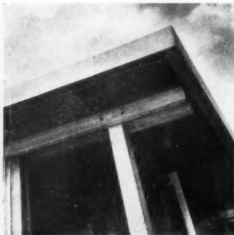
Below left: At corner stanchions in the administration and laboratory block the cladding is set back. Infilling includes asbestos cement panels, beaded in, and vertical cedar boarding, the latter being shop fabricated into panels requiring fixing only. The perimeter paving of the building is generally exposed aggregate concrete with cobbles infilling areas when the cladding has been set back. Below right: in the same position, the column head is exposed, showing the assembly of the main members of the aluminium frame.
