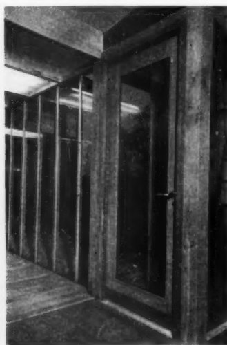
Below left: door frames similarly butt directly up to stanchions, where they are adjacent. Below right: the link to the test shops, fully glazed both sides, punctuates clearly the circulation from one block to the other.
