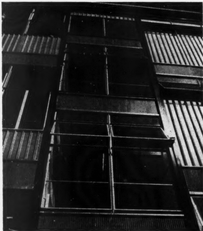
Above prefabricated construction developed by the MOE, Coventry City Architect's Department and Bristol Aeroplane Company using aluminium—Lyng Hall and Whitley Abbey comprehensive schools.
