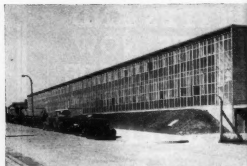
I.C.T. factory at Castlereagh with aluminium curtain walling construction. One extruded section was used to frame the curtain wall at head, sill and jambs. Architects: Smyth & Cowser, F.F.R.I.B.A.
