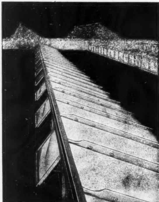
Use of Plyglass shows the saving achieved over conventional roof lighting. Architects: Gotch, Saunders and Surridge, Kettering
