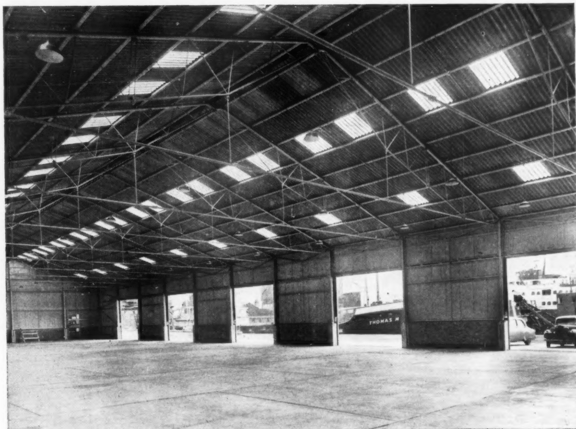
'Arcon' 75 foot span transit building supplied by Taylor Woodrow (Arcon) Ltd., for Dover Harbour Board, Dover, Kent, in which Clear Corrugated 'Perspex' sheet, type 568, has been used for the roof lighting. Consultants: Coode & Partners.
