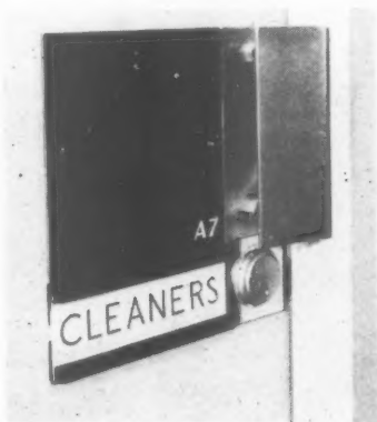
This carefully worked out solution to a door furnishing problem that is usually left to take care of itself is typical of the standard of detailing throughout the building. Attention has been paid to every surface and junction and each item of equipment has been judged in relation to its context. Unfortunately in this case the handle is too sharp at the edges and so close to the jamb that fingers can easily be trapped.
