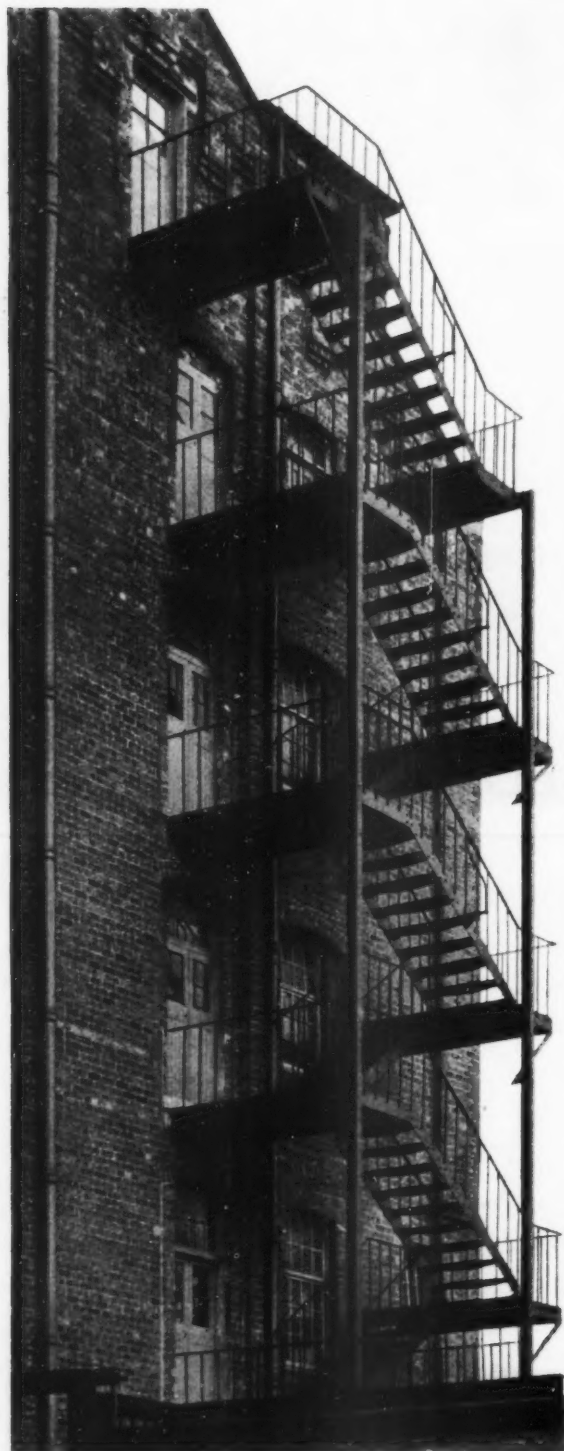
Lion Fire Escape Stairs are made for strength and safety. Available either straight or spiral, they are constructed in steel with cast iron perforated treads and landings. For over sixty years Lion Foundry Co. Ltd. have been supplying and erecting fire-escape stairs for Government Buildings, Local Authorities, Hospitals, Office Blocks, Theatres, etc.
