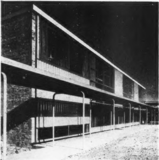
Above: external view of assembly hall. The ground level window lights a store under the stage. The loose pebbles on this side of the covered way form the open top of a land drain. Below: inside the assembly hall, used also as a gymnasium.
