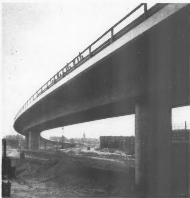
These pictures show a variety of solutions adopted for the elevated road or bridge approach carried on a single row of r.c. columns. Left, from top to bottom: the tramway approach at Mannheim, mushroom-shaped columns supporting a 4-lane highway at Ludwigshafen, and a single carriageway at Düsseldorf. Right, from top to bottom: 4-lane by-pass at Bingen, 4-lane viaduct at Unkelstein, 2-lane approach to Severins Bridge, Cologne, and (below) the experimental Alweg monorail near Cologne.
