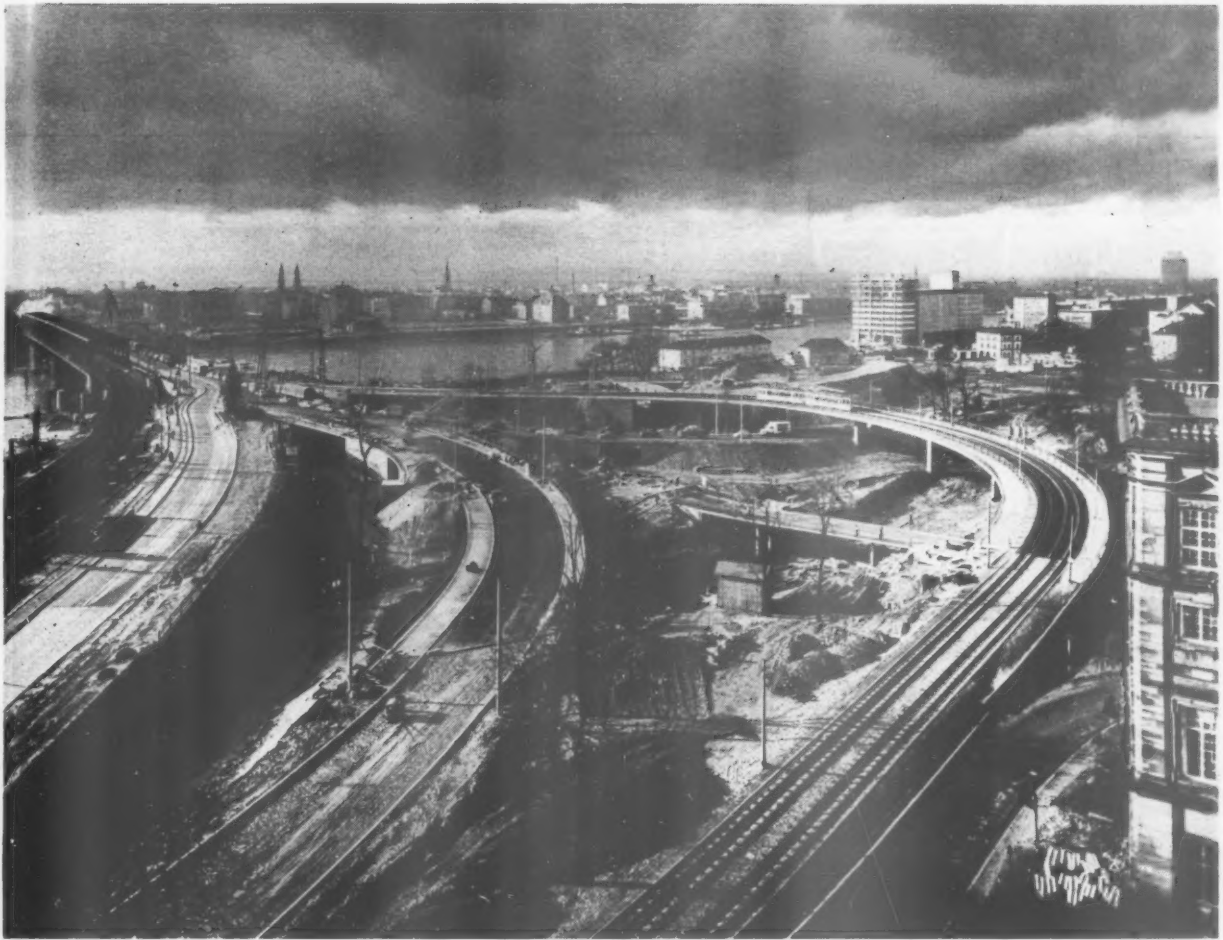
Top: a view of the Mannheim bridge approaches under construction, with Ludwigshaven on the other side of the Rhine, and the separate tramtrack in the foreground. This complex of roads discharges its traffic straight into the streets of Mannheim, whereas in Ludwigshaven the intention is to build one elevated road to carry through traffic out of the city, and another to encircle the central area (see plan, opposite). The smaller pictures show, left, close up of the Mannheim approach and Castle; below, left to right, three views of the Ludwigshaven ramps: (a) tram track entering the town under the elevated bridge approach, (b) lorry emerging from underpass, and (c) the elevated roads left unfinished at the point where the road to the west is to join the inner ring road; the complete scheme is expected to take 10 years.
