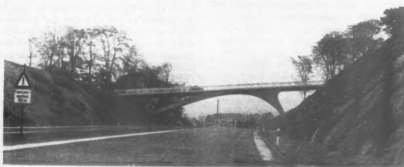
Above, "The Picasso Bridge," near Wuppertal, on the new Wuppertal-Cologne autobahn, showing the use of saplings to bind the embankment before planting. Below, bridge carrying an approach road over the motor road at a Cologne intersection.
