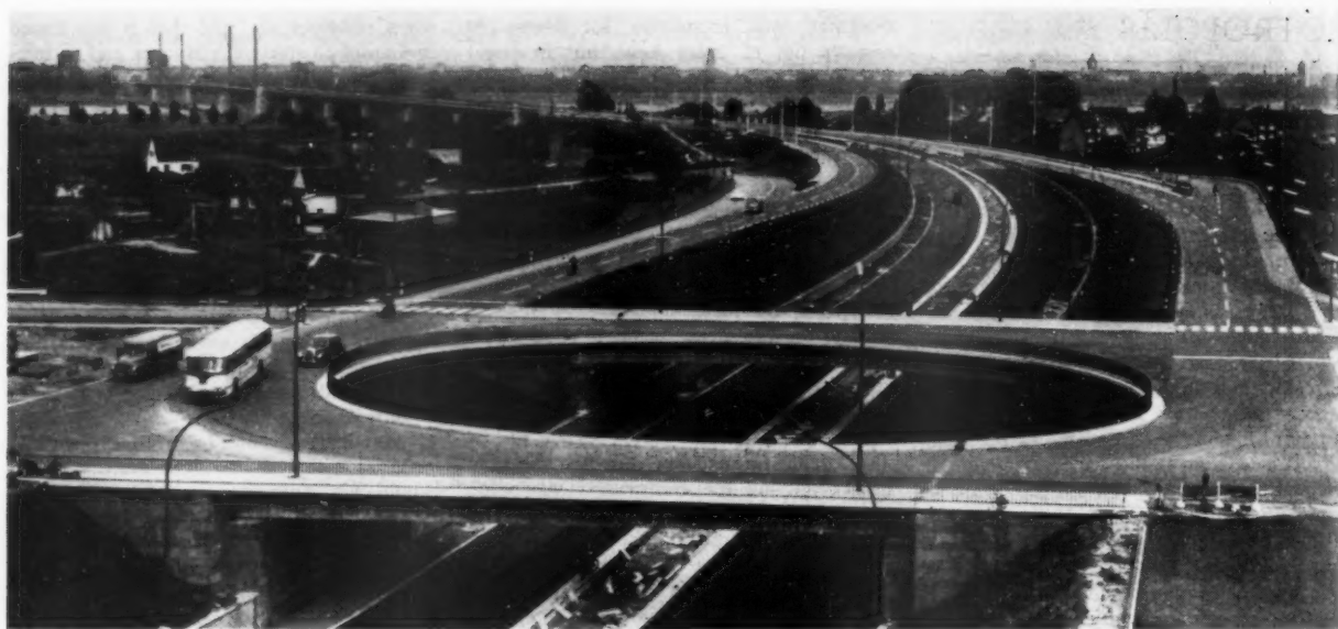
The Seestern flyover roundabout, on the urban motor road linking Düsseldorf (in the background) with the West by the Nordbrücke over the Rhine. This scheme which brings the autobahn system to within two miles of the city centre is more fully illustrated on page 582.
