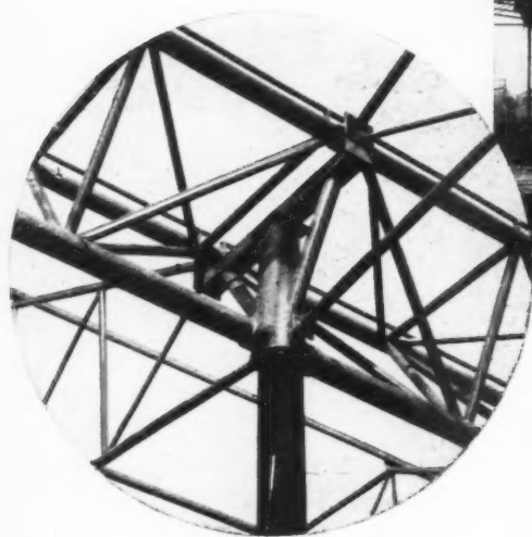
Top: General view of trusses and triangular girders of the tubular steel roof work.
