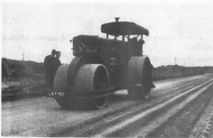
Figs. 1-3. Multi-pass method for mix-in-place soil stabilization. Fig. 1 (top). A rotary hoe with a cement hopper attachment mixes the cement with the pulverized soil. (Note in the previous operation the same rotary hoe but without the hopper, was used to scratch up and pulverize the soil.) Fig. 2 (centre). Water is added to the cement soil mixture. Fig. 3 (bottom). A smooth wheeled roller gives a final surface.
