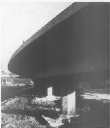
These pictures show a variety of solutions adopted for the elevated road or bridge approach carried on a single row of r.c. columns. Left, from top to bottom: the tramway approach at Mannheim, mushroom-shaped columns supporting a 4-lane highway at Ludwigshafen, and a single carriageway at Düsseldorf. Right, from top to bottom: 4-lane by-pass at Bingen, 4-lane viaduct at Unkelstein, 2-lane approach to Severins Bridge, Cologne, and (below) the experimental Alweg monorail near Cologne.
