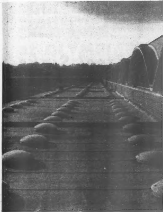
Some of the 180 diffused opal "Perspex" domes installed at the Murphy Radio Factory for the Welwyn Garden City Development Corporation. Architect: C. W. Hutton, B.Arch., F.R.I.B.A. General Contractors: John Laing & Son Ltd.
