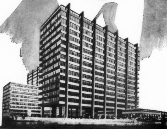
STATE HOUSE. Architects: Trehearne & Norman Preston & Partners. Builders: Tersons Ltd. Electrical Contractors: Rashleigh Phipps & Co. Ltd. G.E.C. equipment: 2-Main Switchboards, Cubicle Pattern, 2-M.W. Switchboards, all 500 volt, Switch and Fusegear, Rising Main Service Units, Alum. Rising Main Busbars, Steel Cable Trunking, Conduit.
