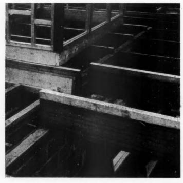
Fig. 7. A detail of the roof construction at St. Michael's, showing laminated timber principal beams.
