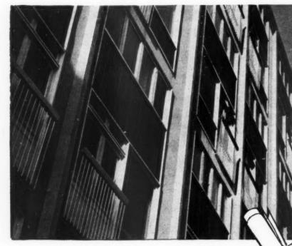
An example of Timber Curtain Walling at Jacobs Wells Flats, Bristol, designed by A. H. Clarke, A.R.I.B.A., A.M.T.P.I., City Architect, Bristol.
