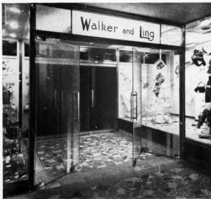
Entrance doors with sidelights at Weston-super-Mare. Special spring and hinge unit with retractable pivot allows door and sidelight to be folded back.
