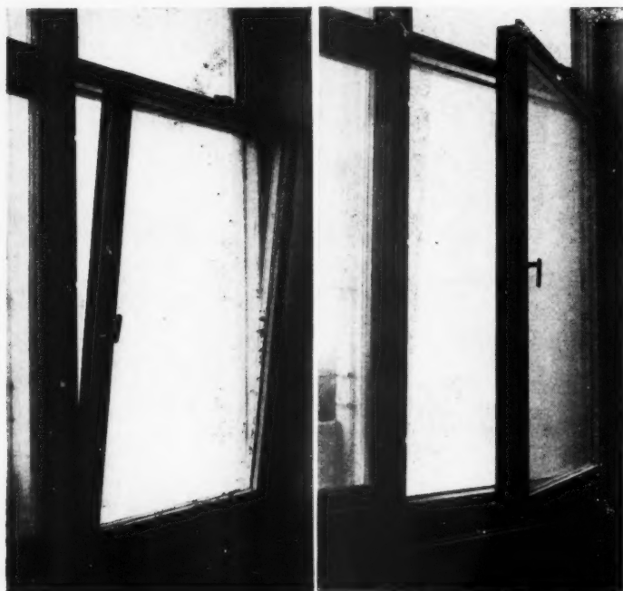
Above and below, fittings designed to enable a window to open inwards—either as a casement or a hopper for night ventilation. Made by Gunther Krebs and Co., Berlin.
