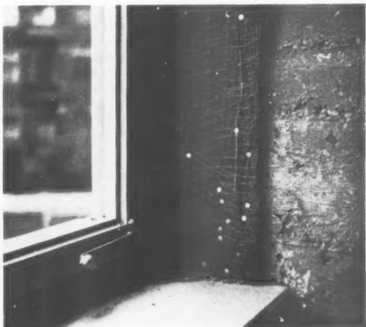
Above, partitioning of lightweight concrete blocks under construction in the recently completed point block by the German architect Gustav Hassenpflug. Note the flat p.v.c. wiring pinned to the wall through the centre, which is plastered over without any extra protection. Below, the end of one of the concrete cross walls in the same block, showing insulating material (bitumen impregnated insulating board) to prevent condensation which might otherwise be caused by the conduction of heat away through the wall at this point.
