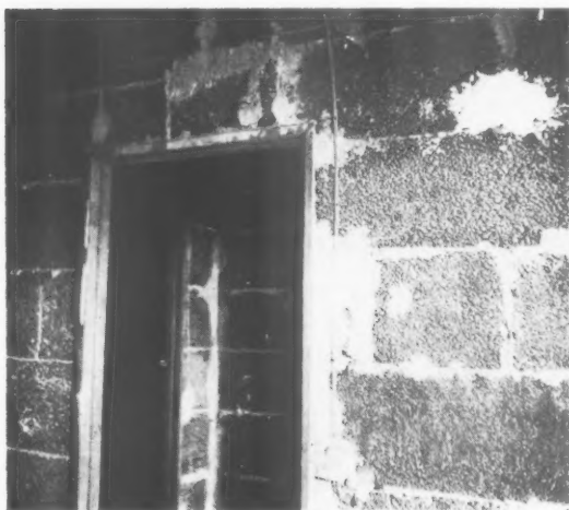
Above, partitioning of lightweight concrete blocks under construction in the recently completed point block by the German architect Gustav Hassenpflug. Note the flat p.v.c. wiring pinned to the wall through the centre, which is plastered over without any extra protection. Below, the end of one of the concrete cross walls in the same block, showing insulating material (bitumen impregnated insulating board) to prevent condensation which might otherwise be caused by the conduction of heat away through the wall at this point.
