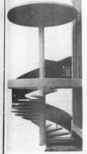
The delicate concrete spiral staircase at the Bonus Pastor Secondary School, constructed by Formcrete Ltd. who were also responsible for the whole of the reinforced concrete frame. Messrs Formcrete is the Reinforced Concrete Specialist Subsidiary Company of W. H. Gaze and Sons Ltd.
