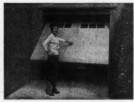
Gear, illustrated on left, represents the best method of operating an overhead-type door, and it requires the minimum space, fixing time and maintenance. An entirely clear threshold is achieved, and both side walls are available for windows and shelves ELLARD "Overdor" Gear is designed for doors from 6ft, to 7ft. 3in. high and up to 200lbs in weight. The door is safely balanced and can be opened and closed with ease.
