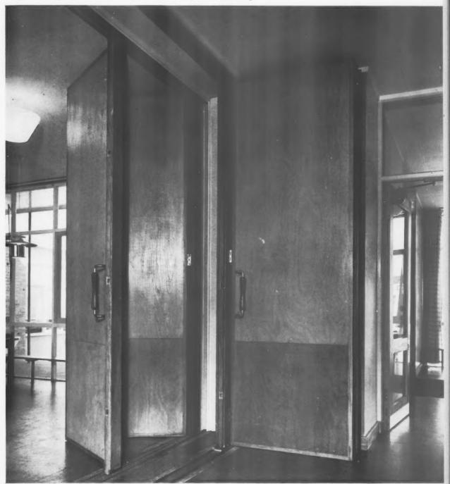
This detail was designed to meet a very common requirement in schools with multi-purpose assembly halls. It has been found in practice that the opening and closing of the doors (and the reversal of the grooved thresholds) takes the caretaker between two and three minutes. The calculated sound reduction for the single leaf is 28 decibels and for the double leaf 40: but actual reductions are 25 and 38, respectively.
