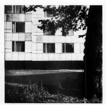
Alvar Aalto's celebrated block faced with very smooth concrete panels made with expanded clay aggregate and imported specially for this building. The panels are a creamy grey colour which make the building a pleasant contrast to the more highly coloured buildings surrounding it. A number of the panels have discoloured and crazed but this has not as yet detracted from its good appearance.
