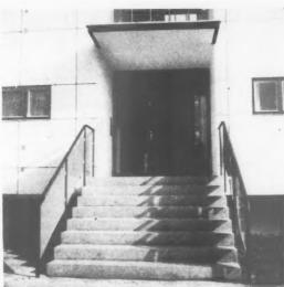
Above and below: the low block by Professors Luckhardt and Hoffmann. Facing panels of white "Eternit," a popular Continental asbestos board having a hard polished surface. The general effect is good. These panels were stuck to the wall but have had to be fixed with screws as well (seen in the joints) to satisfy the local building inspector. The balustrades are filled with red plastic sheets.
