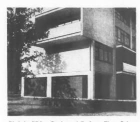
Block by Walter Gropius and Professor Ebert. Balcony fronts in white enamelled steel. Walls of concrete painted white, infilling panels under windows rendered light grey. Balcony soffits and rear walls painted bright blue with balcony sides orange. This block is exceptional in having metal windows. See AJ Working Detail, October 31, 1957.
