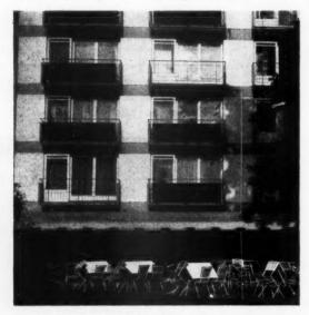
Seventeen-storey point block by Müller-Rehm and Siegmann. Storey height smooth precast concrete facing panels of 5-cm. lightweight concrete cast on to 5-cm. woodwool used as permanent shuttering to a 20-cm. in-situ concrete wall. Painted cream with grey bands at floor levels and royal blue canvas wind shields fixed to some of the balcony railings. This block, containing small flats for single people, has a restaurant on the ground floor, with a yellow awning.
