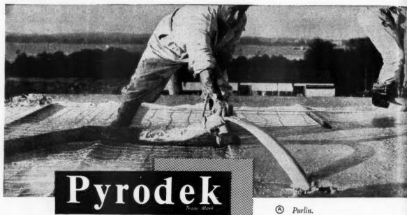
An entirely new lightweight roof construction in which Gypsum Concrete is poured into place to a depth of 2 in. on bulb tee sections, formboard and reinforcing fabric to form an incombustible roof economical for areas of over 500 square yards.
