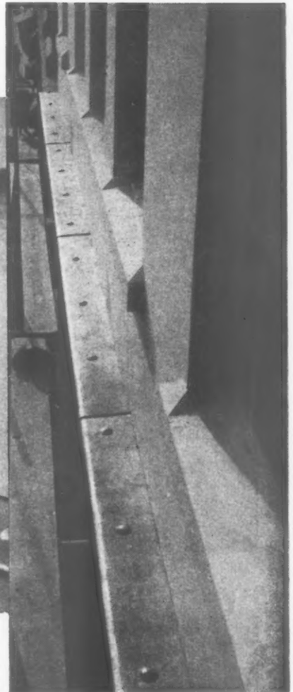
A typical example of lead weatherings for stone-faced buildings. New office building, London W.1 Architect: H. G. Sumner, L.R.I.B.A.
