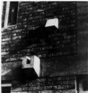
Brick and Concrete at Ham; a detail of wall, floor-slab, ventilator and gargoyle from a new flatted development at Ham Common by James Stirling and James Gowan.
