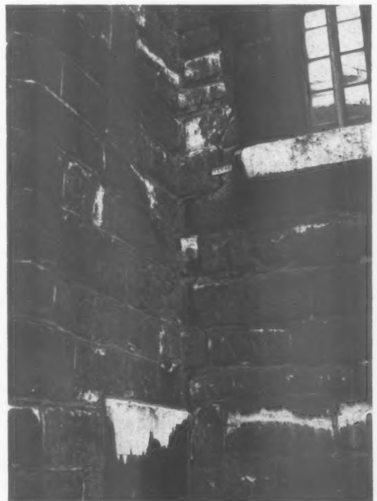
Cement tell-tale on a crack in a re-entrant angle at Fulham Palace. (Photograph by courtesy of MOW.)
