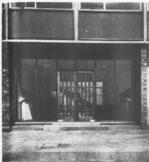
The entrance has a glazed screen, of teak, across the full width of the bay and teak double doors. Below, another view looking outwards from the entrance hall.
