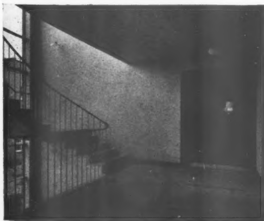
The main stairwell looking along the nurses' home corridor on the first floor. The acoustic tile ceilings are painted pale blue (BS 7-077). The staircase is finished in terrazzo with non-slip nosings and plastic handrail to balusters. The floor is of grey marble lino tiles with black strip inserts. The corridor doors are of mahogany with ribbed aluminium kicking plates.
