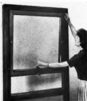
2. Releasing the casement
