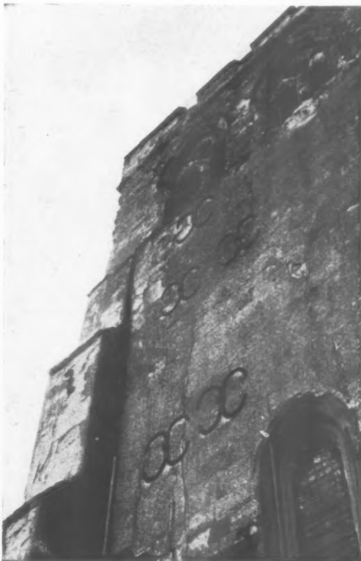
Vertical cracks in a church tower caused by bell-ringing.
