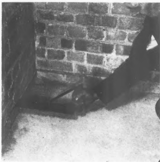
Cutting horizontal damp-proof courses. Above, by means of a light pneumatic saw; below, using an electric saw mounted on a supporting frame.
