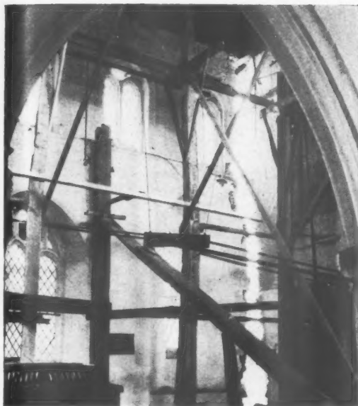
Left, internal and, right, external view of the rectification of a leaning aisle wall by the use of winches. Orby Church, Lincs. (Architect, John E. MacGregor.)
