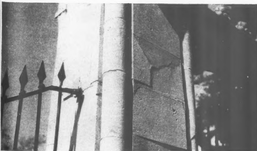
Not all faults are due to neglect. The rusting of iron fixings has caused this damage.
