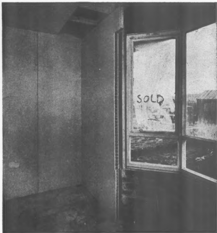
'Paramount' DRY Partition used as an internal lining in a Modern House.
