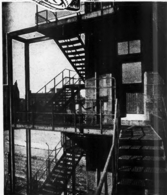
Lion Fire Escape Stairs are made for strength and safety. Available either straight or spiral, they are constructed in steel with cast iron perforated treads and landings. For over 60 years Lion Foundry Co. Ltd., have been supplying and erecting fire-escape stairs for Government Buildings, Local Authorities, Hospitals, Office Blocks, Theatres, etc.
