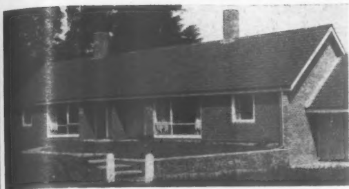
Two typical houses, from the south-east. There are three slightly different types of house in the scheme, with different internal arrangements of bedrooms, bathroom and kitchen space, but externally they are alike, with pitched roofs covered with dun-coloured clay pantiles, Ewhurst multi-coloured facing bricks and clad in parts with deep red sand-faced club-headed tiles.
