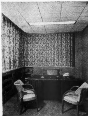
Director's office: Insulated double-wall Compactite partitions, veneered and polished light oak. Fittings designed and constructed by Compactom. Acoustic tile ceiling with flush lighting.
